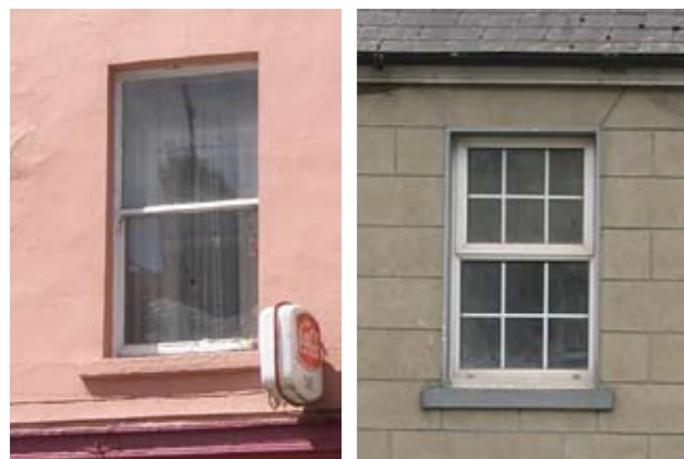
Lime based roughcast and plain ruled and lined renders
