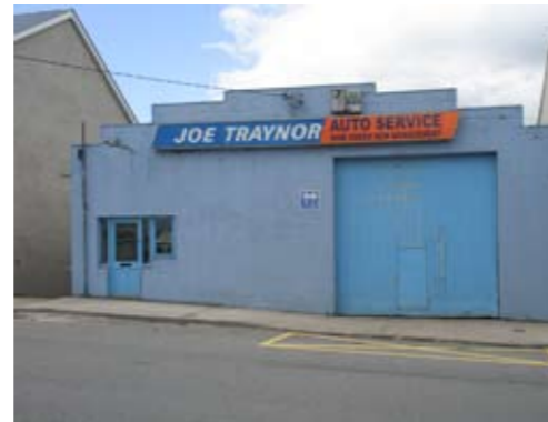
Garage on Main Street Lower
