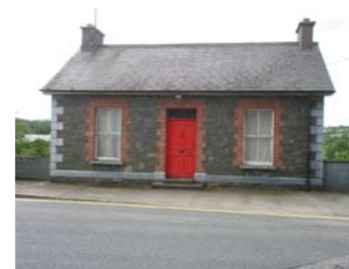
Gas Manager's House, Hall Street
