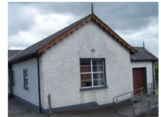
Irish Church School, Church Street
