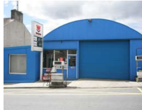
Garage on Main Street Lower
