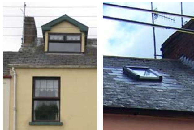
Inappropriate dormer window and roof light
