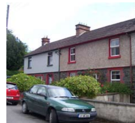
Terraced housing at Church Street
