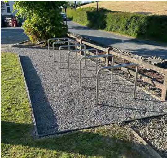
Figure 37 - Lisdoonan Recreation & Development Association – installation of bicycle racks
