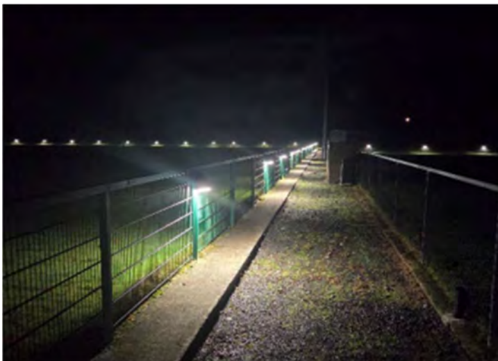
Figure 38- Aghadrumsee St. Marcetan's CLG Fermanagh – Installation of low-level LED lighting at walking track
