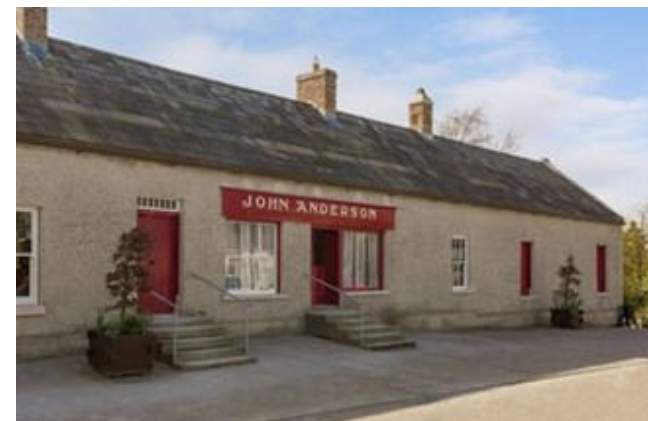
Drum: Andersons Vernacular Refurbished Protected Structure
