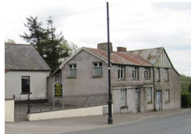
Drum—Vacant Dwellings adjoining the Gospel Hall
