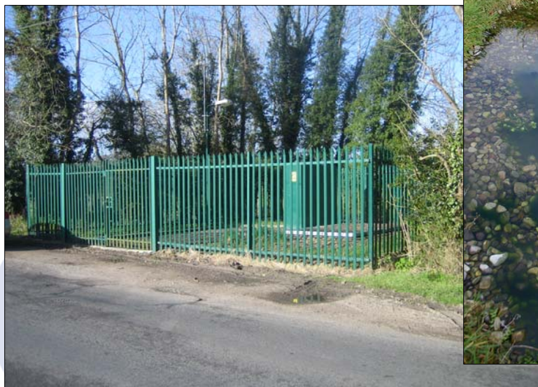
Public Water Supply: Borehole
