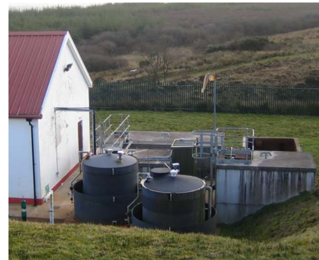
Tydavnet GWS water treatment plant
