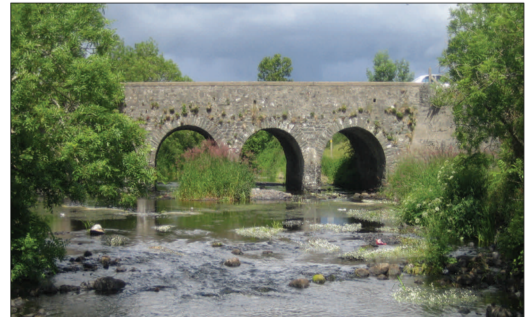
The Fane River system supplies water to Churchill-Oram Group Water Scheme, Inniskeen Village, Newry and Dundalk
