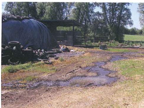
Poor structures and lack of collection facilities may result in water pollution
