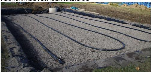
Photo No 3: Sand Filter under construction
