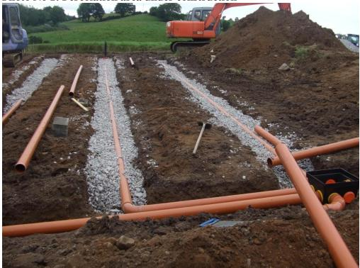
Photo No 1: Percolation area under construction
