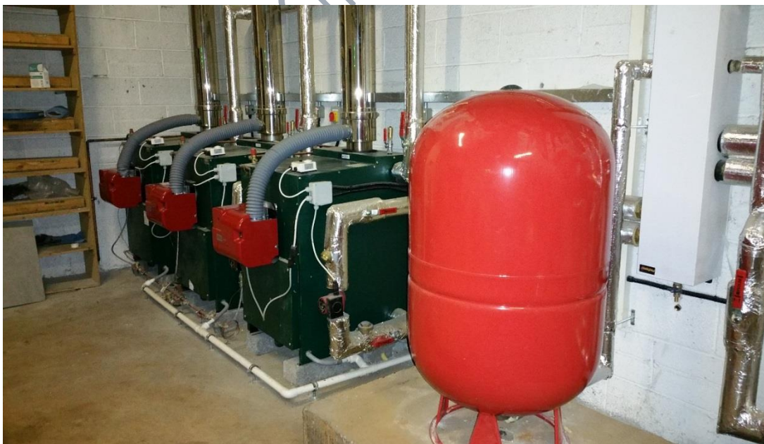
New High Efficiency Oil Burner installed in Council HQ under BEC 2017 – Glen Offices
