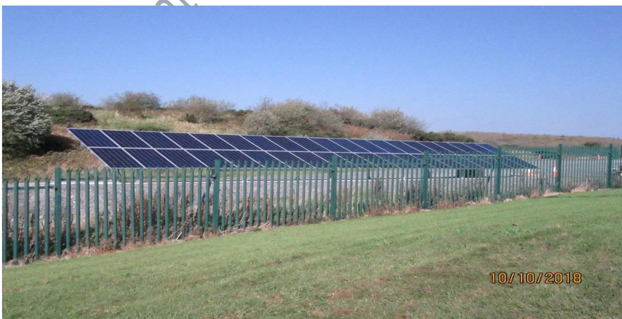
Solar PV Installation at Scotch Corner landfill provided under the 2018 BEC Scheme
