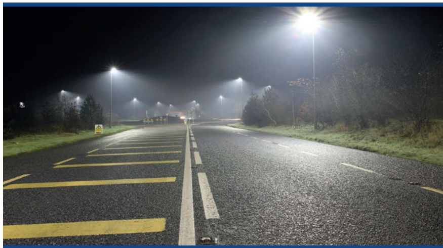
Figure 43 - MCC Public Lighting Retrofitted with LED's.
