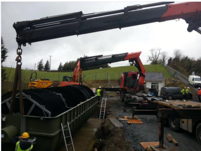
Threemilehouse WWTP Upgrade - Installation RBC
