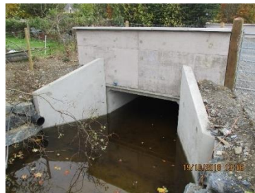
Drumbroagh Bridge R180
