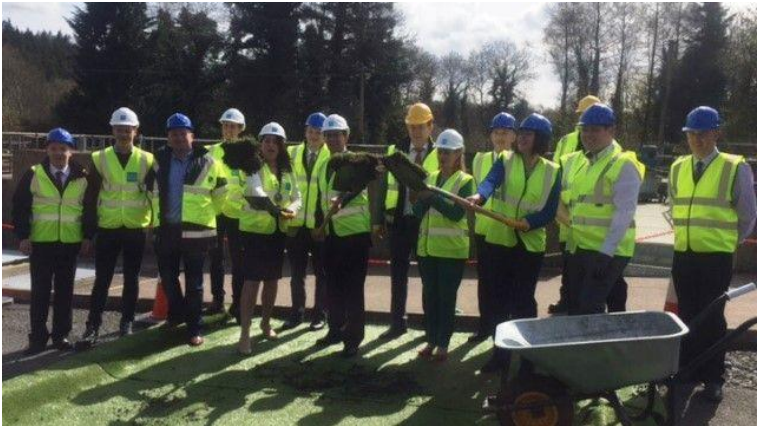
Turning the sod on Castleblayney Waste Water Treatment Plant Upgrade
