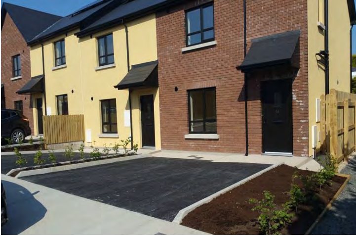
Figure 9. Completed Units secured in Carrickmacross under Part V Agreement
