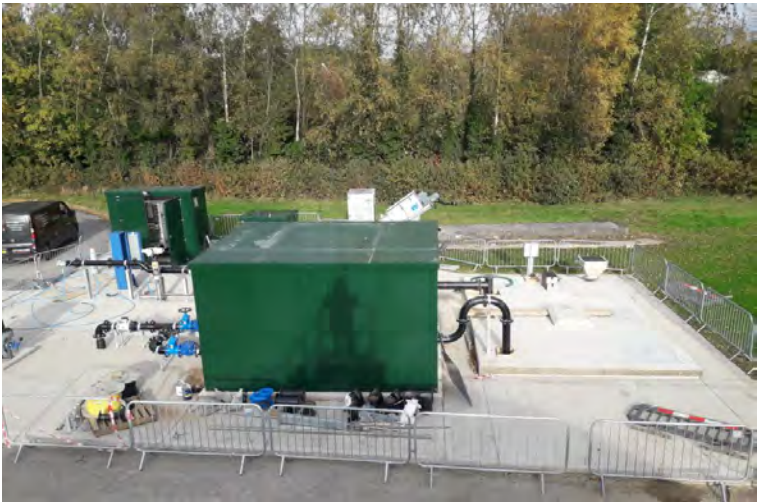
Imports works upgrade Monaghan WWTP
