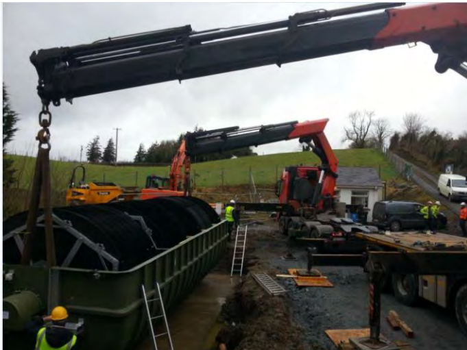
Threemilehouse WWTP Upgrade - Installation RBC
