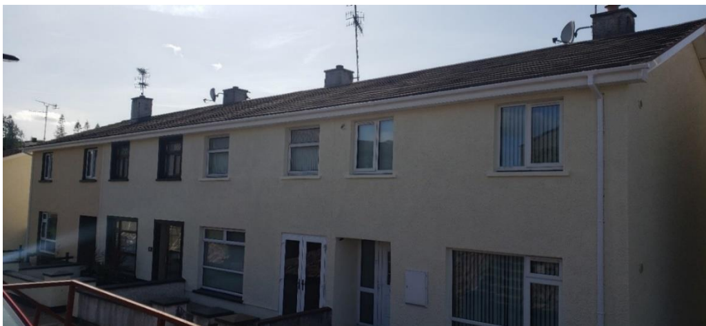
Houses with roof works and painting completed.
