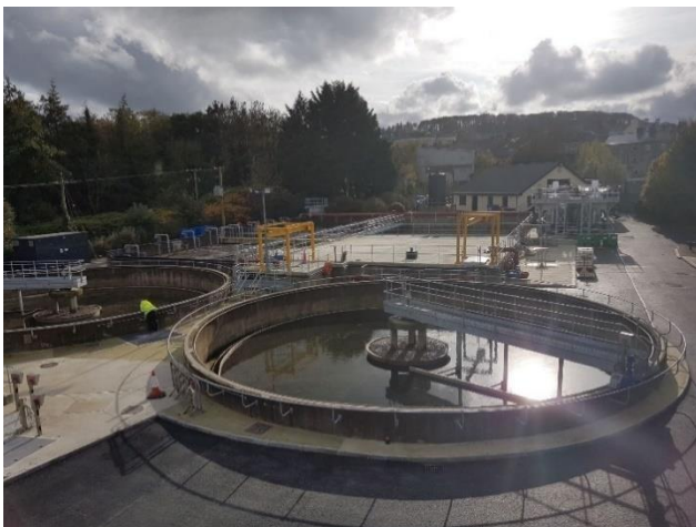
New Waste Water Treatment Plant Castleblayney – Cost €4.4m
