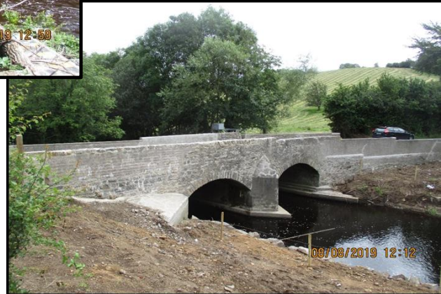
Faulkland Bridge, Post Rehabilitation works, Summer 2019.
