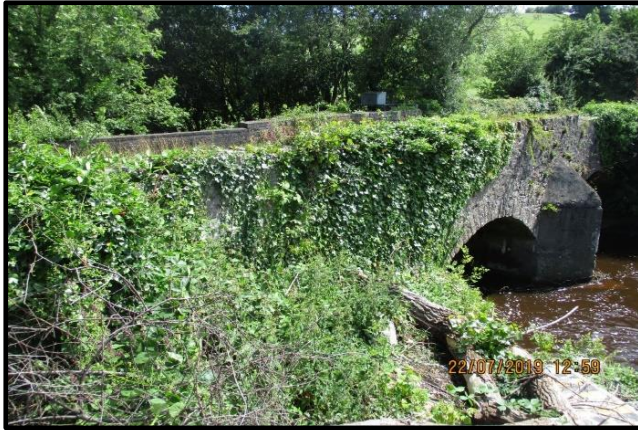
Faulkland Bridge, Pre-works Summer 2019.
