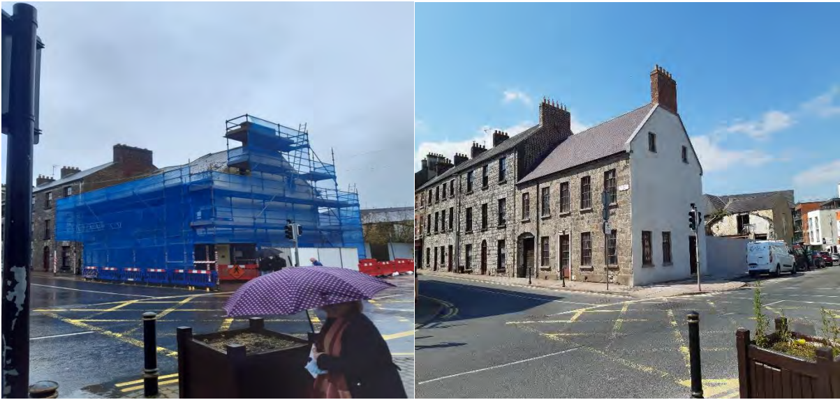
4/5 Mill Street – Emergency Stabilisation Works
