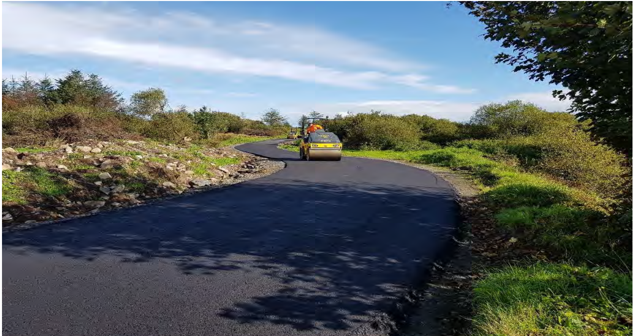
Local Improvement Scheme works at Drum
