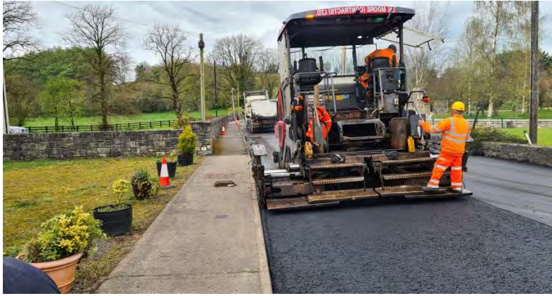
Figure 1: 2021 overlaid under the Road Restoration 2021 program
