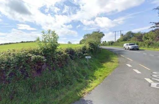
R188 Drummuck before works
