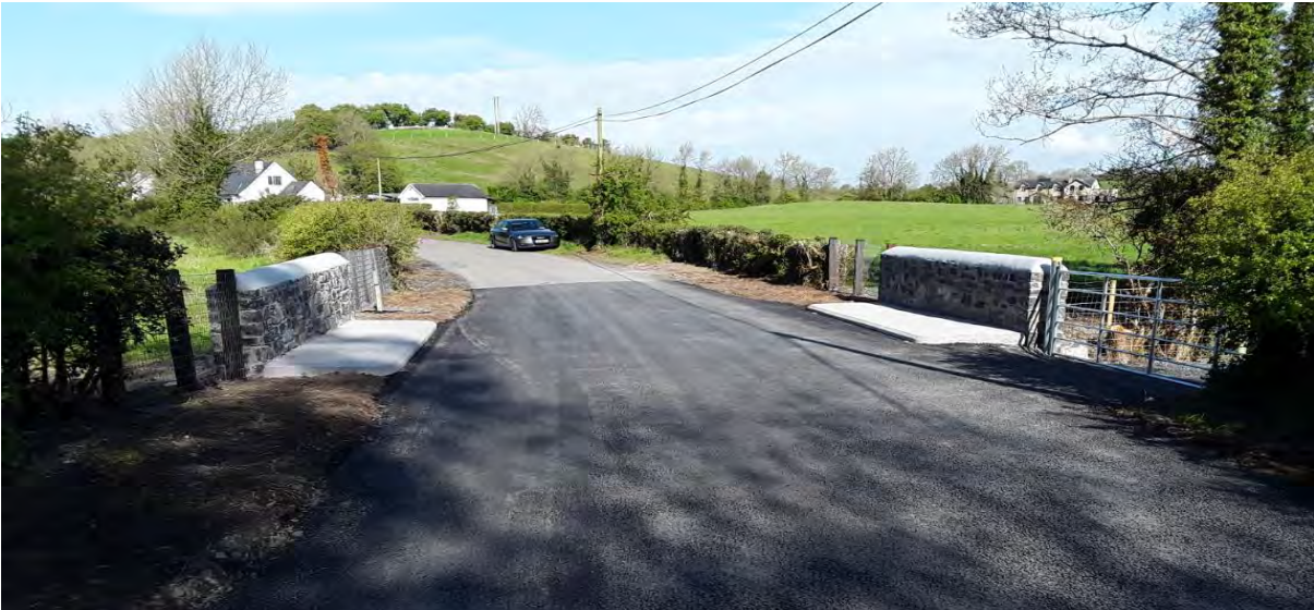
Rehabilitation works at Scarvy - L-2201
