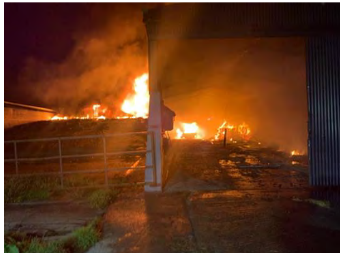
Fire-fighters extinguishing a Diesel Laundry Plant fire Aug 2021
