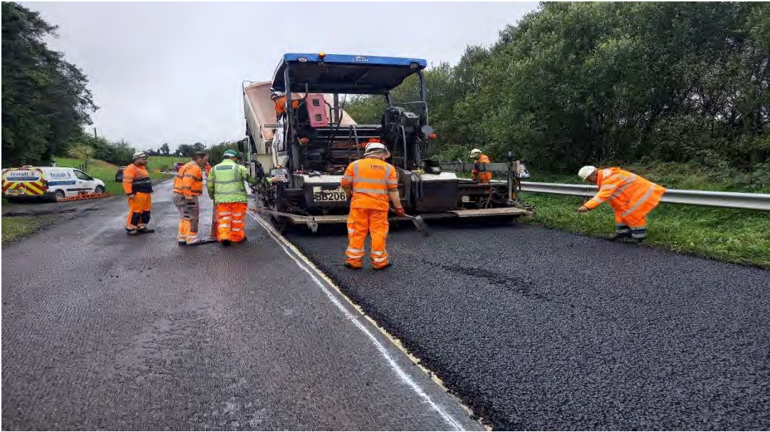
Resurfacing works at N54 Clonlura
