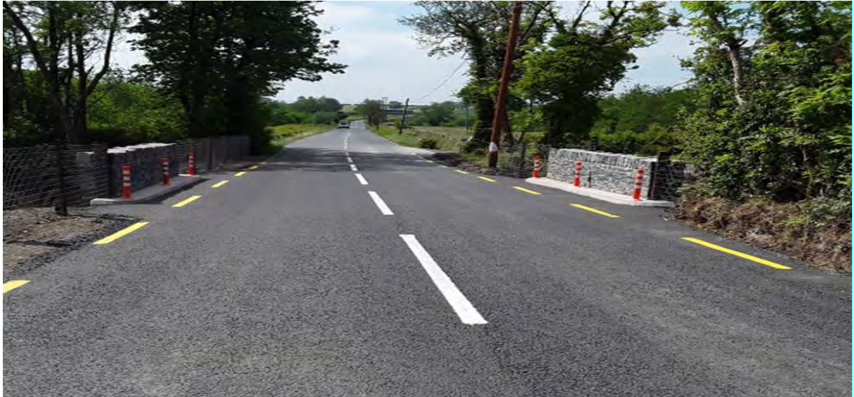
Rehabilitation works at Listroar Bridge – R-184
