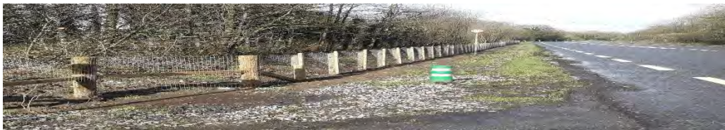
Fencing works at Lough Oony.
