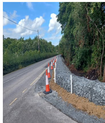
Figure 3 & 4: Verge Slippage Reinstatement Works on the R213 (Before and after photos).
