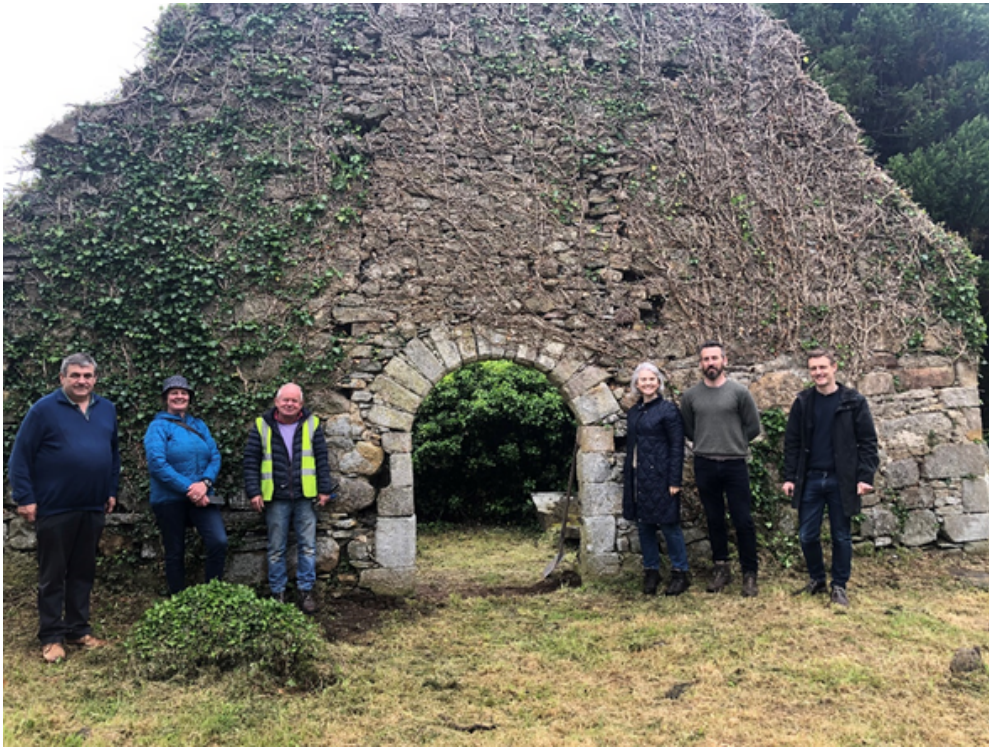
The team at Errigal Truagh medieval church before conservation works commenced.
