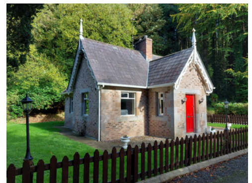
Repaired Finials at Newbliss Gate Lodge, Rossmore, Monaghan
