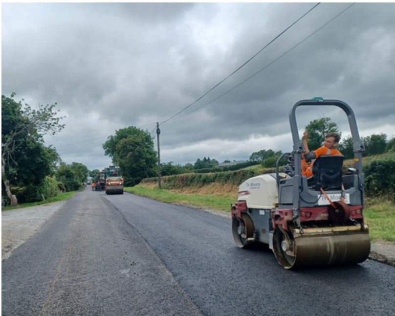
Figure 7: Restoration Improvement Grant. Surface Overlay strengthening works of the LP-3421 Scotch Corner.
