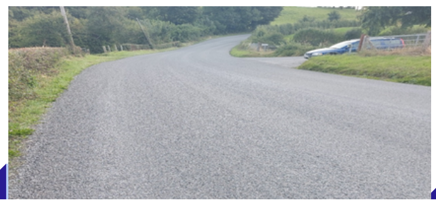
Figure 5: Restoration Maintenance Grant. Surface Dressing works of the R-187.
