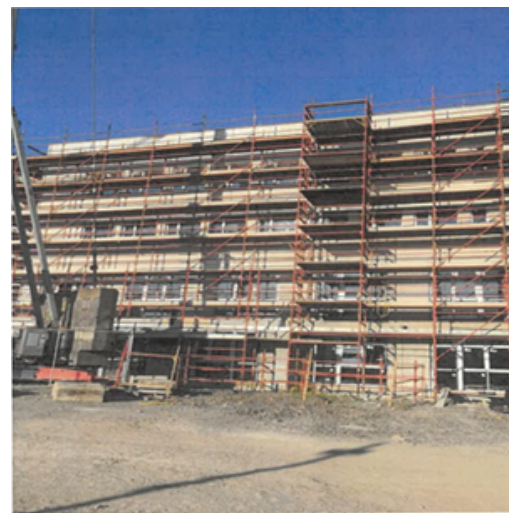
The Ridge” Enterprise Hub, McGrath Road, Castleblayney
