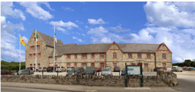
The Workhouse, Carrickmacross
