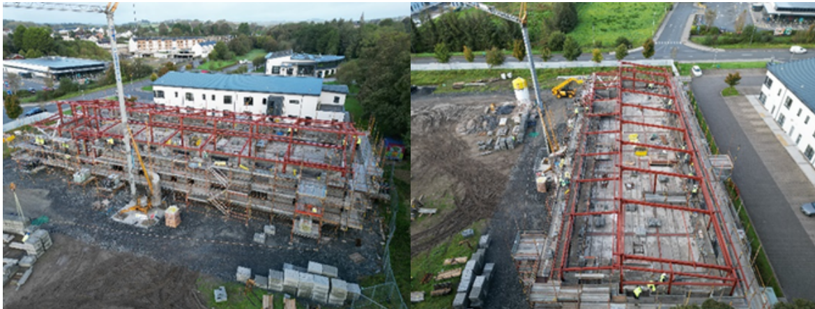
Construction of the new C: Tek II Co-working Enterprise Hub, Carrickmacross
