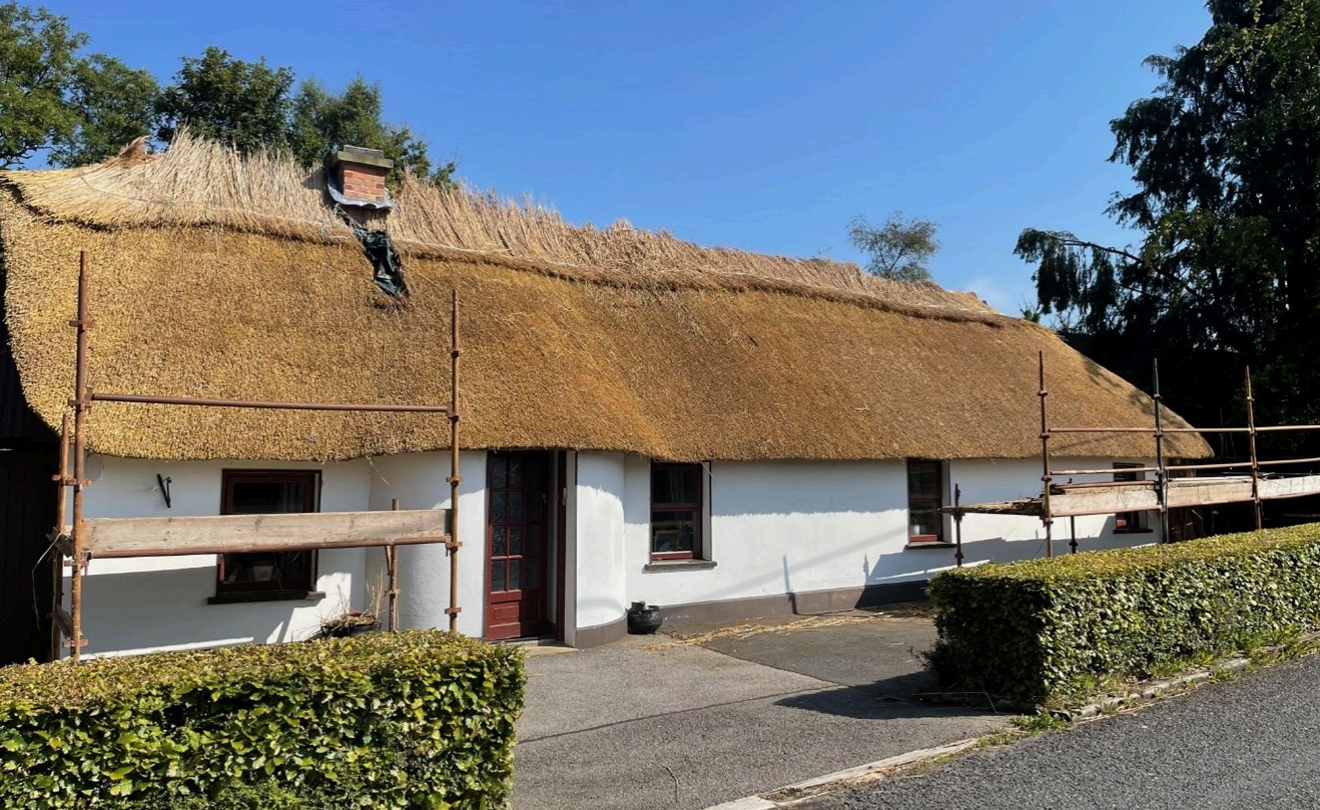
Thatching work reaching completion at Grennan's Cottage
