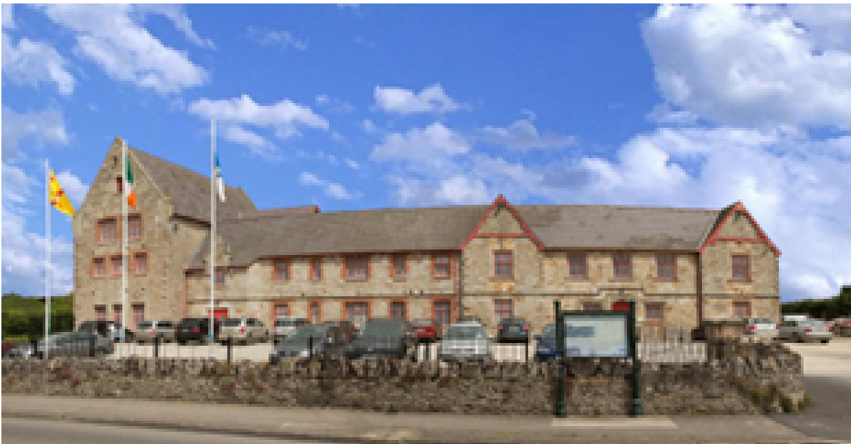
The Workhouse, Carrickmacross
