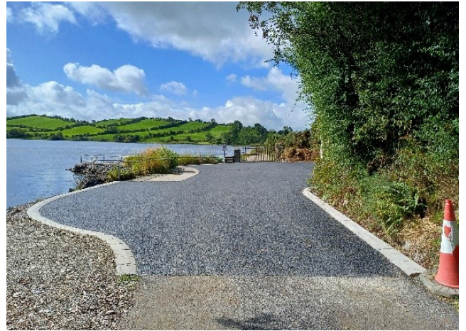
Upgrade of jetty and car parking facilities at Lough Nagarnaman
