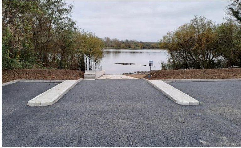
New jetty and slipway at Rahans Lake
