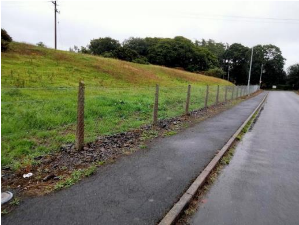
Figure 6.5.8: Roadside hedge removed and replaced with fencing. (MN1008)
