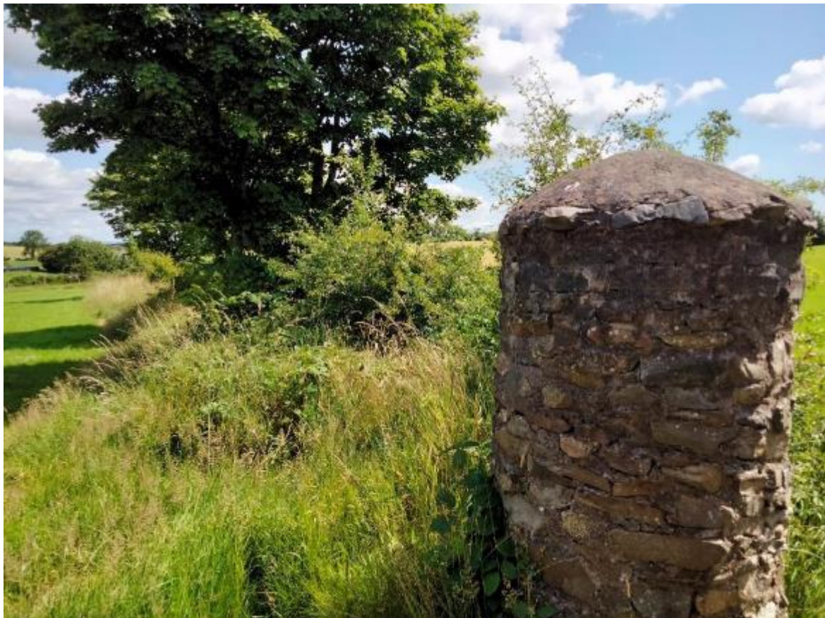
Figure 6.3.5.: Old stone pillar at MN0909 on the old Dundalk-Enniskillen railway tracks.
