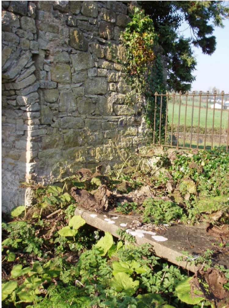
Fig. 31 The interior of the Anketell plot is overgrown and needs clearing
