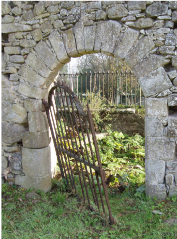
Fig. 13 Gate into the Anketell plot. This needs urgent removal and refurbishment
