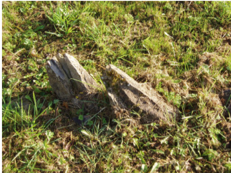
Fig. 44 Trip hazard. These stones, the base of damaged grave-markers, should be left in situ
