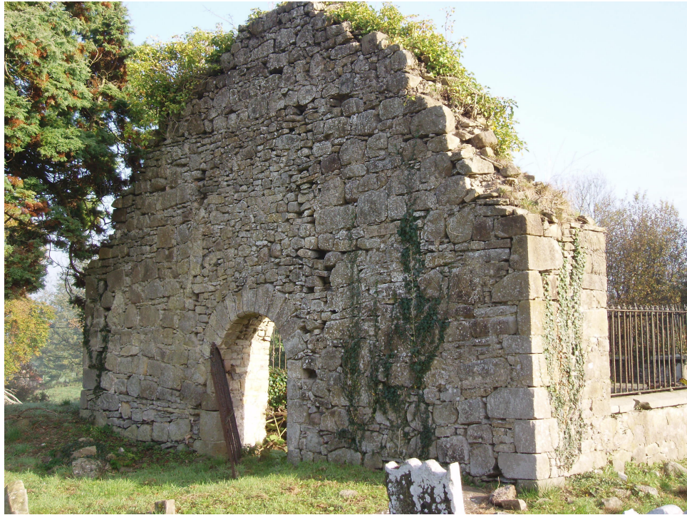
Fig. 1: The west gable of the church at Errigal Truagh
