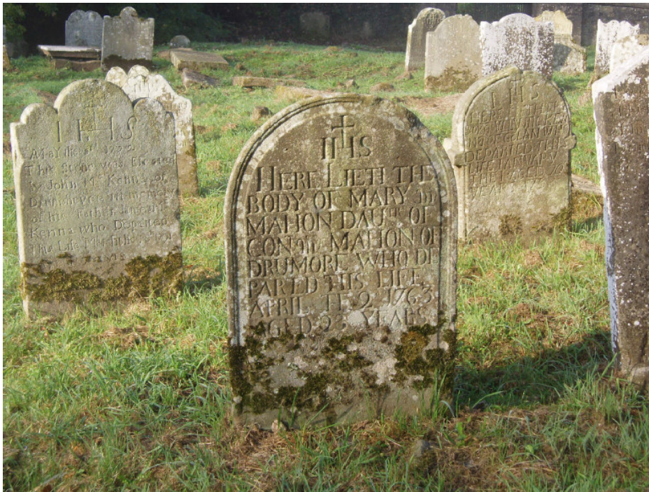
Fig. 25 Moss and lichen cover some of the gravestones. Expert advice should be sought on whether this will eventually cause damage to the stonework
