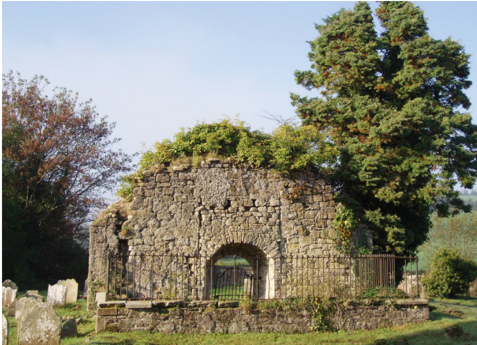
Fig. 18 The fir tree to the north of the church gable will eventually cause problems without regular pruning
