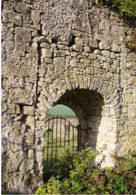
Fig. 14 Inner elevation of doorway through the west gable of the church
