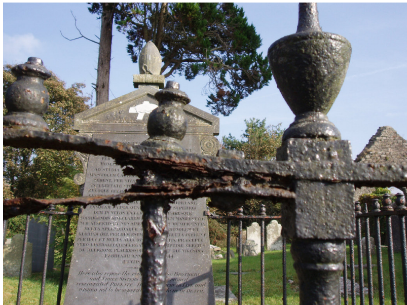
Fig. 29 Much of the ironwork encircling the enclosures is in poor condition
