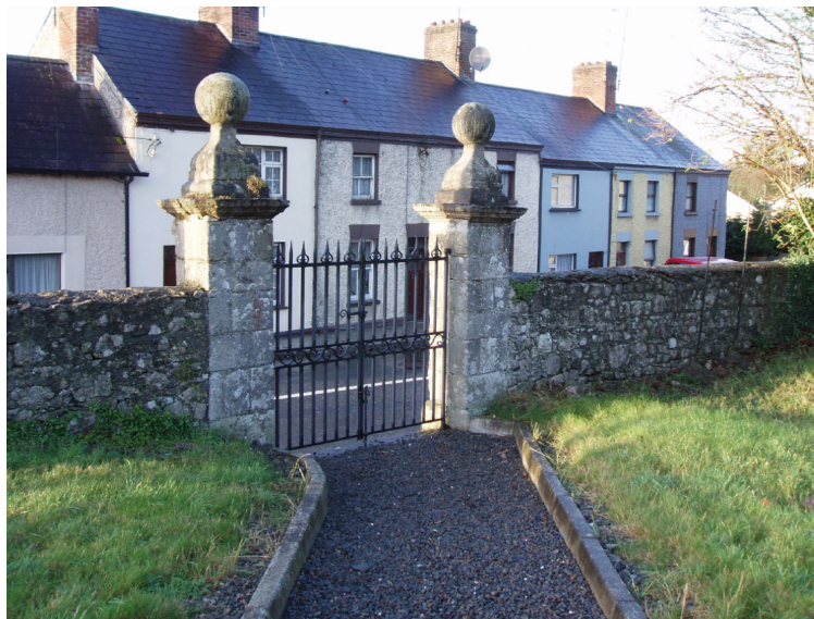
Fig. 46 The entrance gate to the site is in good order
