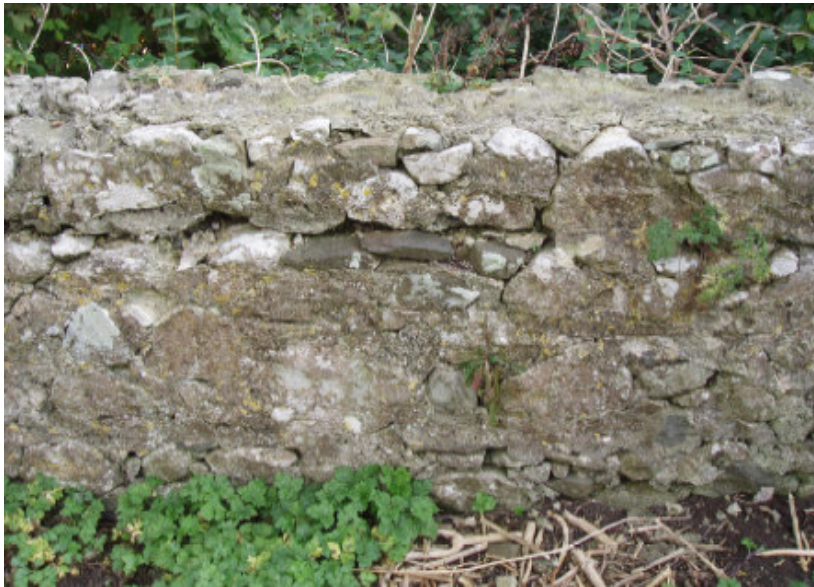
Fig. 44 Detail of the south wall
