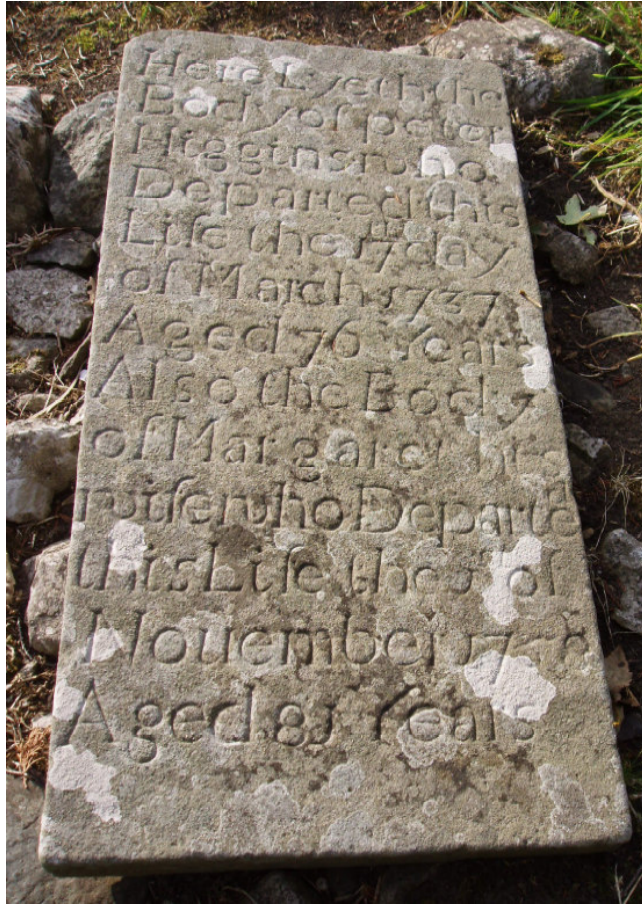
Fig. 28 The fine inscriptions on some of the grave markers are susceptible to damage from weathering
