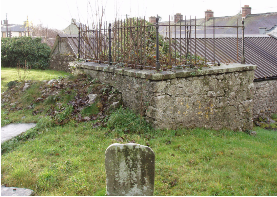
Fig. 35 Enclosure 4, with its corbelled entrance to the underground vault situated to the left of the picture
