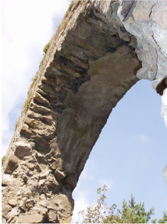
Fig. 17 The underside of the main nave window
