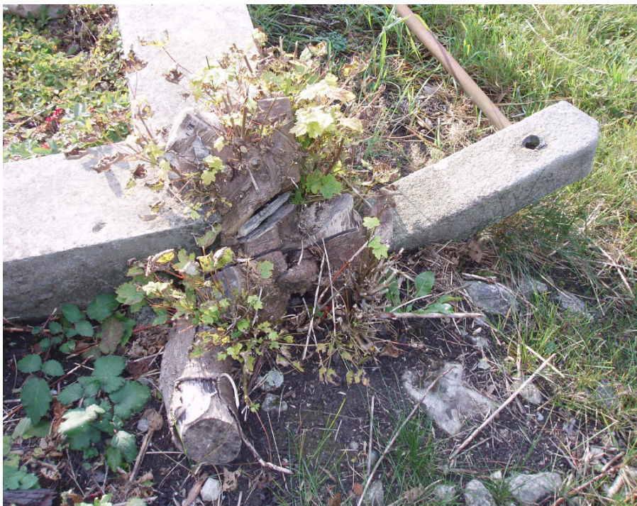
Fig. 32 Detail of the damaged corner post to Enclosure 1
