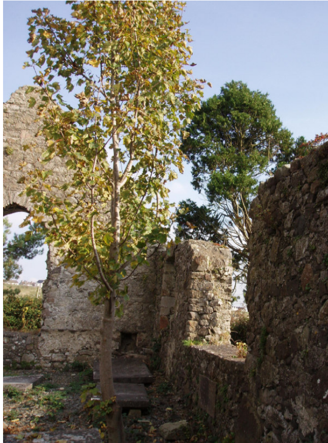
Fig. 16 A tree within the nave needs removal before its roots damage surrounding fabric and underlying archaeological deposits
