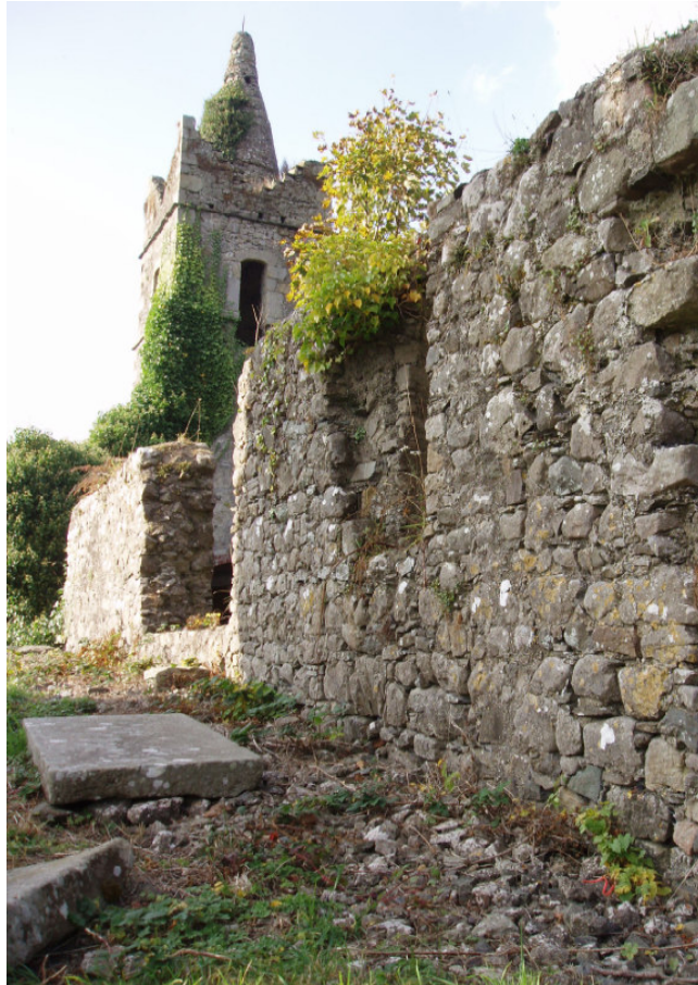
Fig. 13 The south wall of the church
