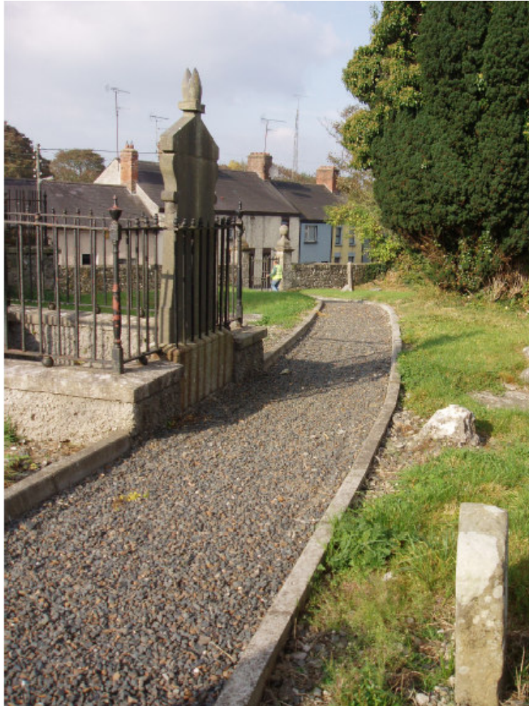
Fig. 23 Although a surfaced path is sympathetic to the church's urban setting, the concrete kerbstones are out of keeping
