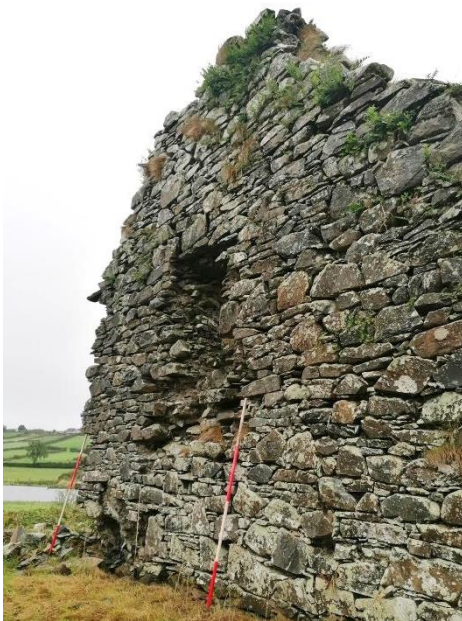
Plate 31 (L): West elevation, note severe collapse on the NW corner and high window Plate 32 (R): Western Elevation, note collapse around the high window
