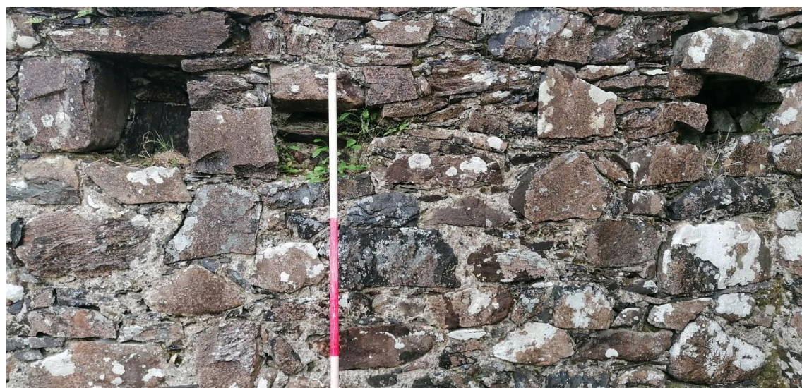
Plate 30: Inner face of south wall, towards the western side. Three beam-holes or empty slots that once held corbel stones for a wooden gallery
