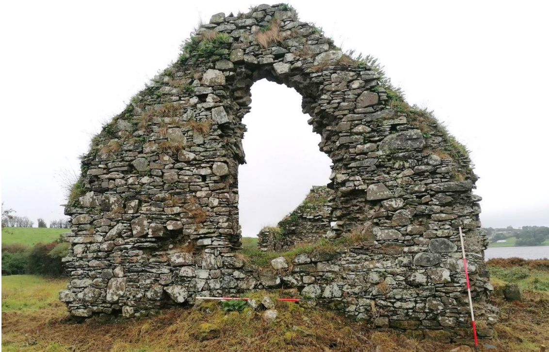
Plate 21: Eastern Elevation (exterior), note the collapsed window and heap of stones at the base, the original window edge and partial arch can be seen along the southern (left) side of the window
