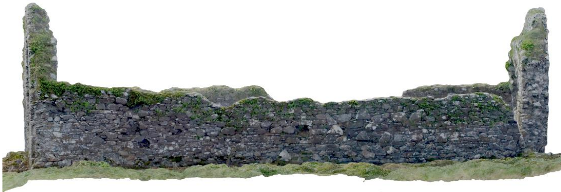
Plate 3: 3D image of north wall
