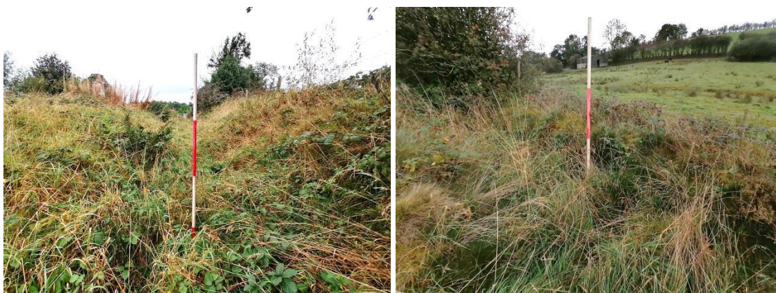
Plate 45 (L): Wide internal ditch to east of graveyard, bank on left, graveyard and chapel on left, facing north Plate 46 (R): Narrow and shallow ditch and bank to SW of graveyard, facing SW
