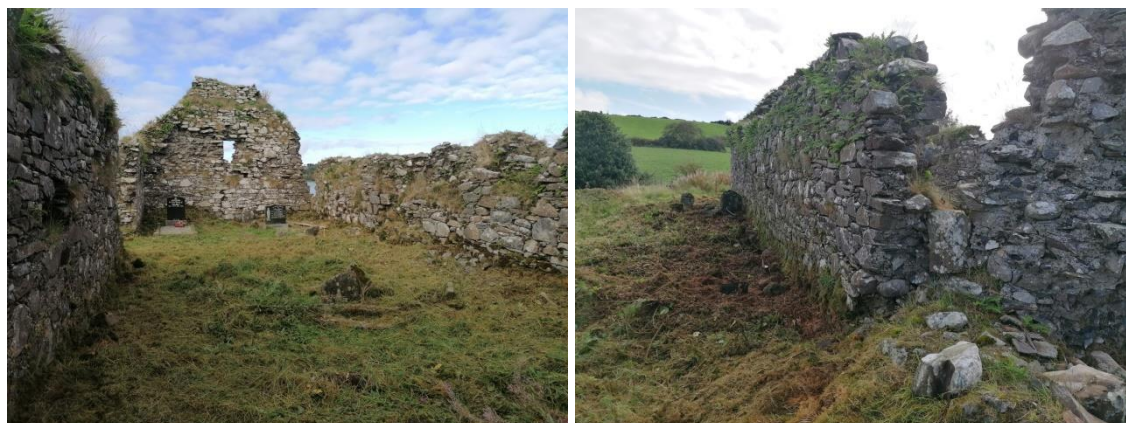
Plate 19 (L): Landscaping work completed, western interior of chapel, Facing W
