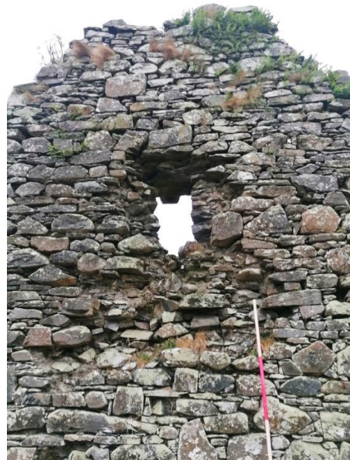
Plate 31 (L): West elevation, note severe collapse on the NW corner and high window Plate 32 (R): Western Elevation, note collapse around the high window
