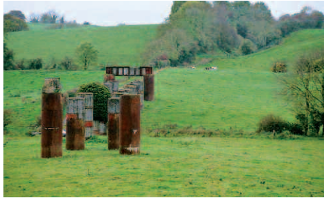
REMAINS OF BALLYNURE VIADUCT
