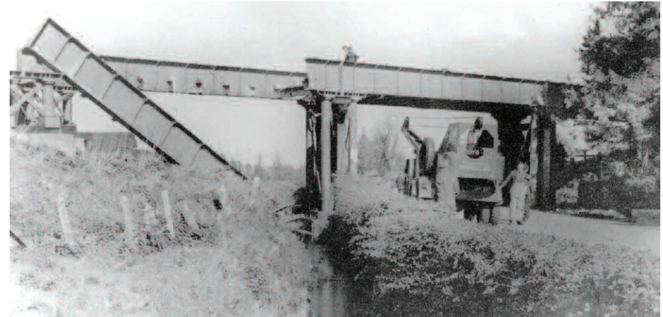
DISMANTLING A RAILWAY BRIDGE MID 1960's
