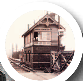
CLONES EAST SIGNAL HOUSE, c. 1910.
