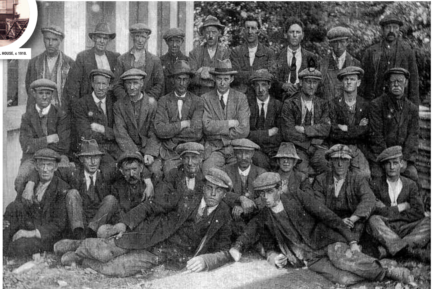
WORKERS AT CLONES STATION - MID 1930's
