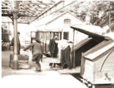
UNLOADING FISH, BALLYBAY 1958
