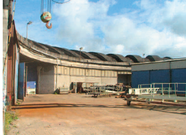
CLONES ENGINE SHED TODAY
