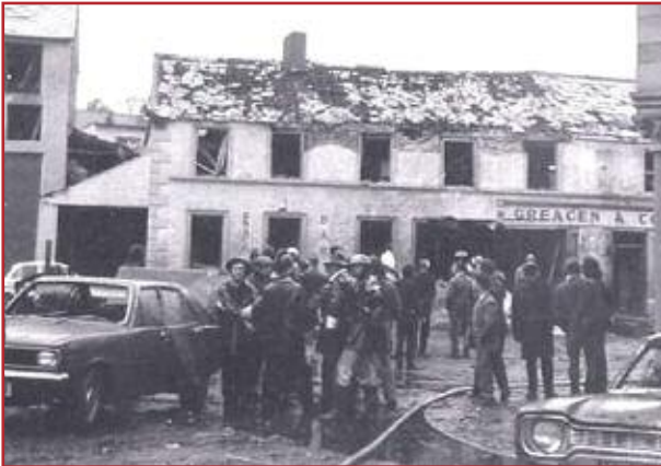
Roof Damage to Greacen's Bar after Monaghan Bomb
