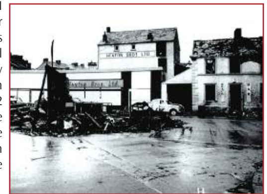
Roof Damage to Greacen's Bar after Monaghan Bomb
