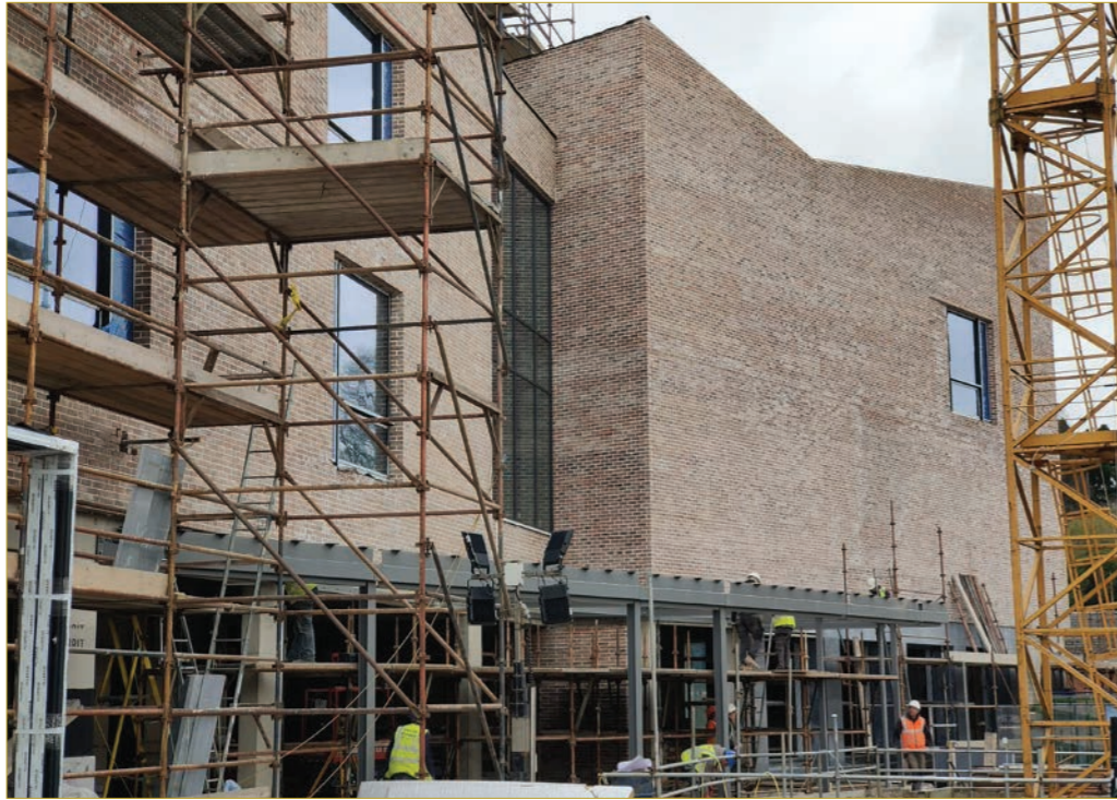
The exterior of the museum-end of the building
