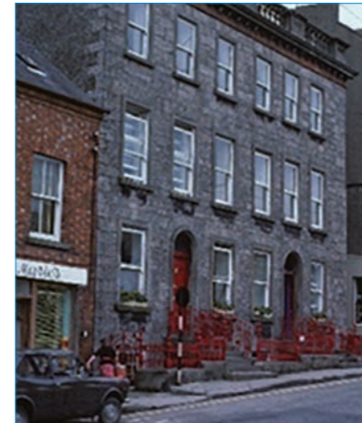
1-2 Hill Street in the 1970s when used as offices for the County Council.
