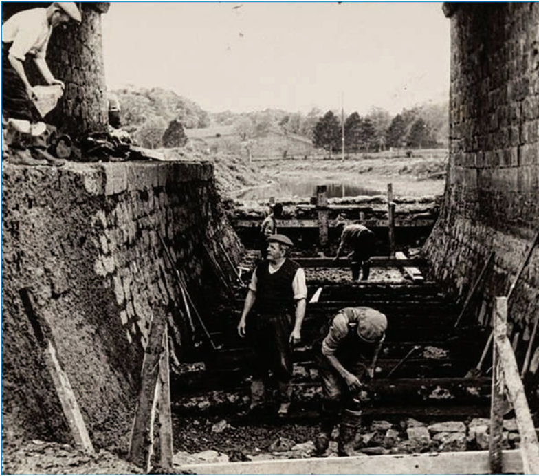
The removal of the canal bridge near Clones c. early 1960's
