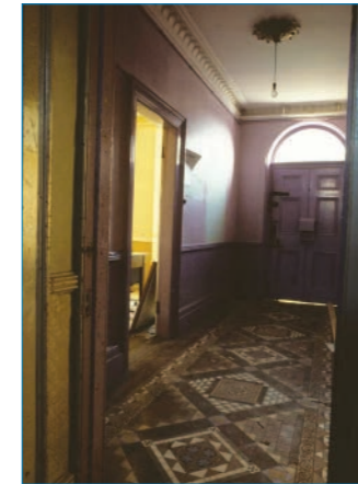
The building undergoing renovations showing the entrance hall with tiled floor.
