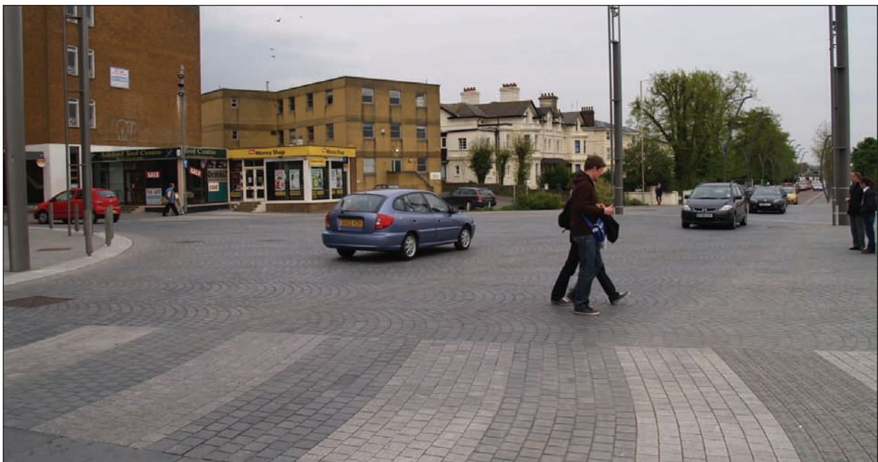
Figure 4.49: Shared surface junction in Ashford, Kent, UK, carries significant amounts of traffic and challenged conventions regarding traffic volumes along shared surfaces. An informal zebra crossing has also been marked adjacent to the junction to provide a place for less confident pedestrians to cross.
