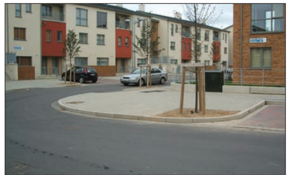
Figure 4.75. Example from Ballymun, Co. Dublin (top) and Leixlip, Co. Kildare (bottom) where kerb build-outs and contrasting materials are used to separate and define bays of parking from the vehicular carriageway, reduce corner radii and facilitate planting or landscape treatments.
