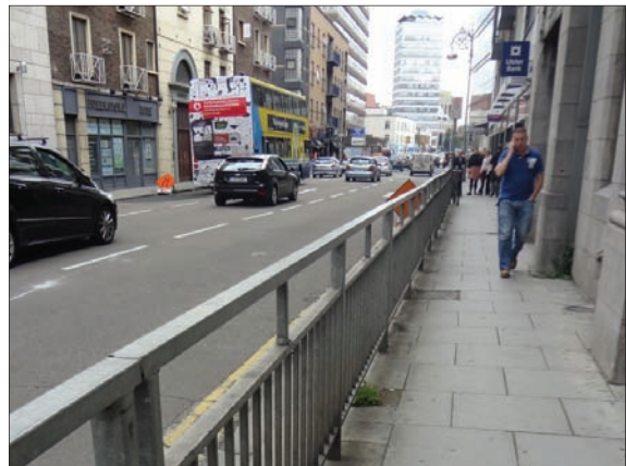
Figure 2.10: Guardrails can create a hazard for cyclists, reduce footpath widths and give rise to feelings of constraint and restriction to pedestrians.
