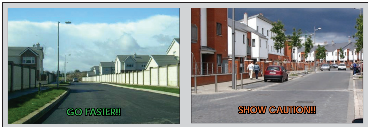
Figure 2.14. The elimination of access and frontage along roads (top) was introduced to reduce risk, but it serves to encourage speeding.
