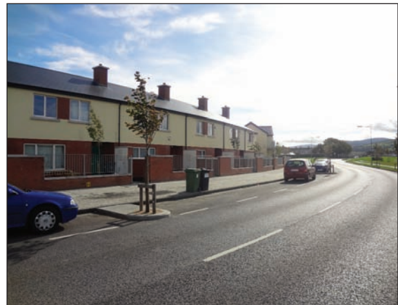
Figure 4.77: Example from Fettercairn, Co. Dublin where a ‘distributor’ style road was narrowed by adding bays of parallel parking as part of a package of works aimed at calming traffic and improving the sense of place.
