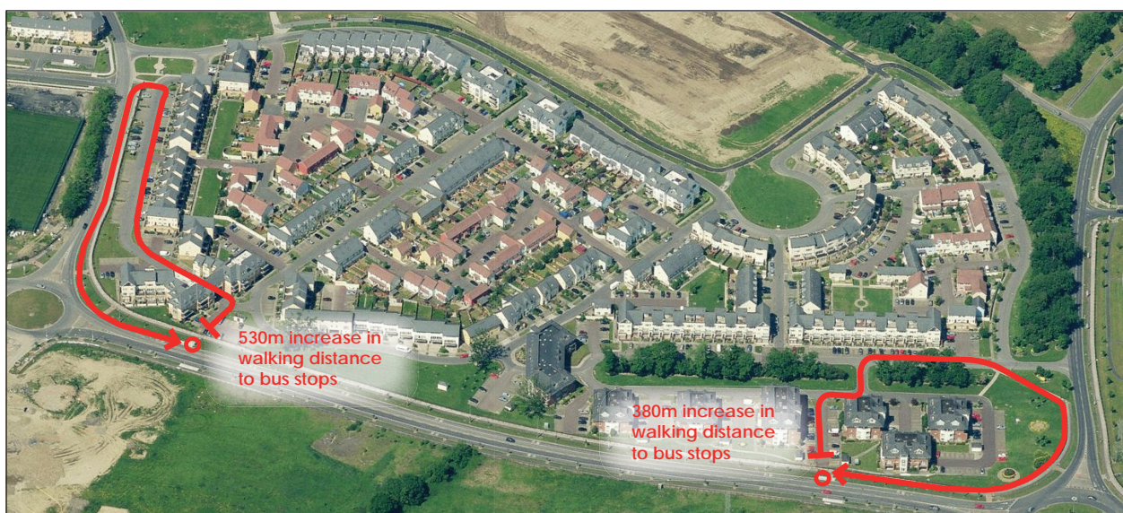
Figure 2.7: Example of a 'neighbourhood cell' located within a 'distributor road' network. A long fence separates the Cell from the Distributor Road. A number of openings in the fence were initially planned to provide access to bus stops. These were removed at the request of residents due to safety concerns, significantly increasing walking distances to bus stops (base image source: www.bing.com/maps ).
