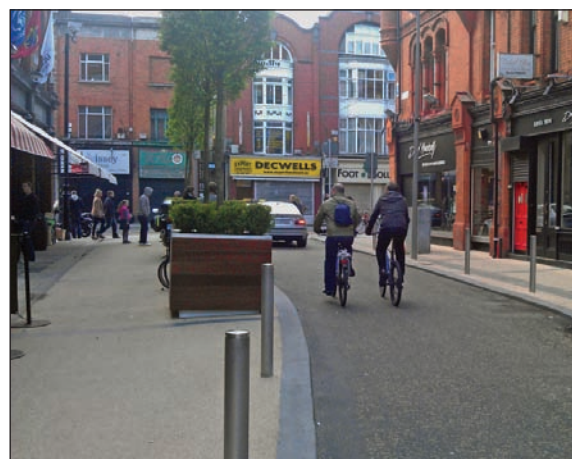
Figure 4.26: Fade Street, Dublin City Centre. To reduce the overall cost of work in remodelling the street, lower budget materials such as HRA with coloured aggregate chips and epoxy resin bound surfaces were used on the carriageway and footpath, respectively.
