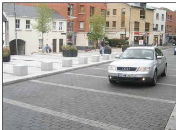
Figure 4.57: Example from Chapelizod, Co. Dublin, where the carriageway has been paved adjacent to a square in a village centre to add value to place and calm traffic in an area of higher pedestrian activity.
