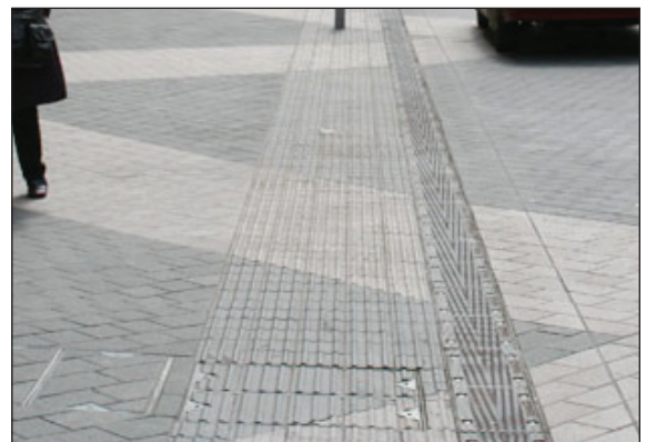
Figure 4.74: Example of a drainage channel on Exhibition Road, London. The kerb line indicates an area of pedestrian refuge and is used to guide the visually impaired.
