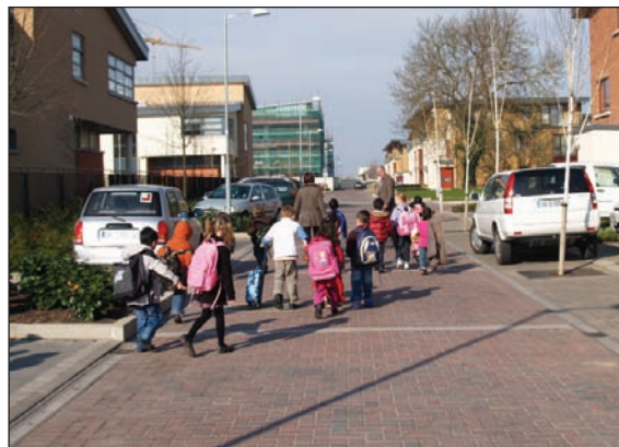
Figure 4.56: Example from Adamstown, Co. Dublin of a shared surface 'homezone' adjacent to a school. Paving materials, combined with embedded kerbs encourage a low speed shared environment.
