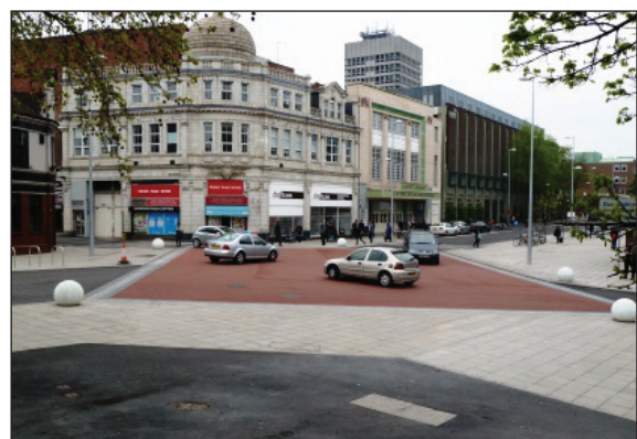
Figure 4.62: Example from Coventry, UK of a shared surface uncontrolled junction. The level of traffic using the junction would normally warrant some form of control, however, its traffic calmed nature allows for drivers to communicate with each other and pedestrians to establish movement priorities (image source: Hamilton-Baillie Associates).
