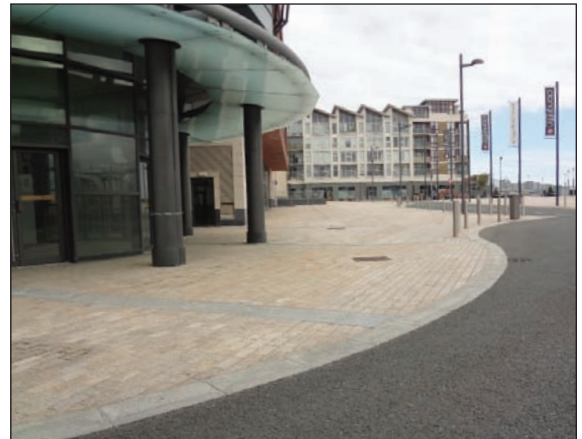
Figure 4.73: Example from Clongriffin Co. Dublin, where the footpath, kerb line and vehicular carriageway are at the same level. Whilst pedestrian and vehicular space are still clearly defined, a greater sense of shared space is still created.
