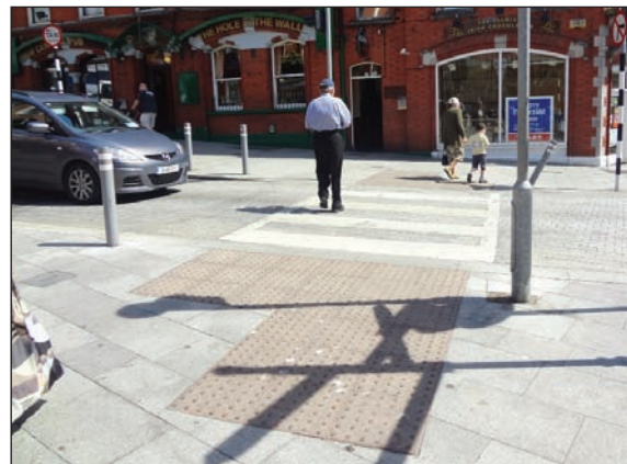
Figure 4.24: Example from Drogheda, Co. Louth, of red tactile paving at a zebra crossing which has been toned down to balance the degree of contrast with higher specification materials.
