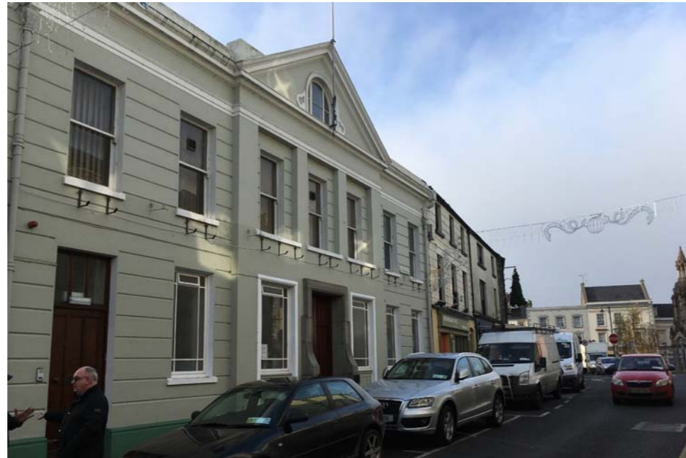
Fig 2.9 Town Council Offices, Dublin Street
