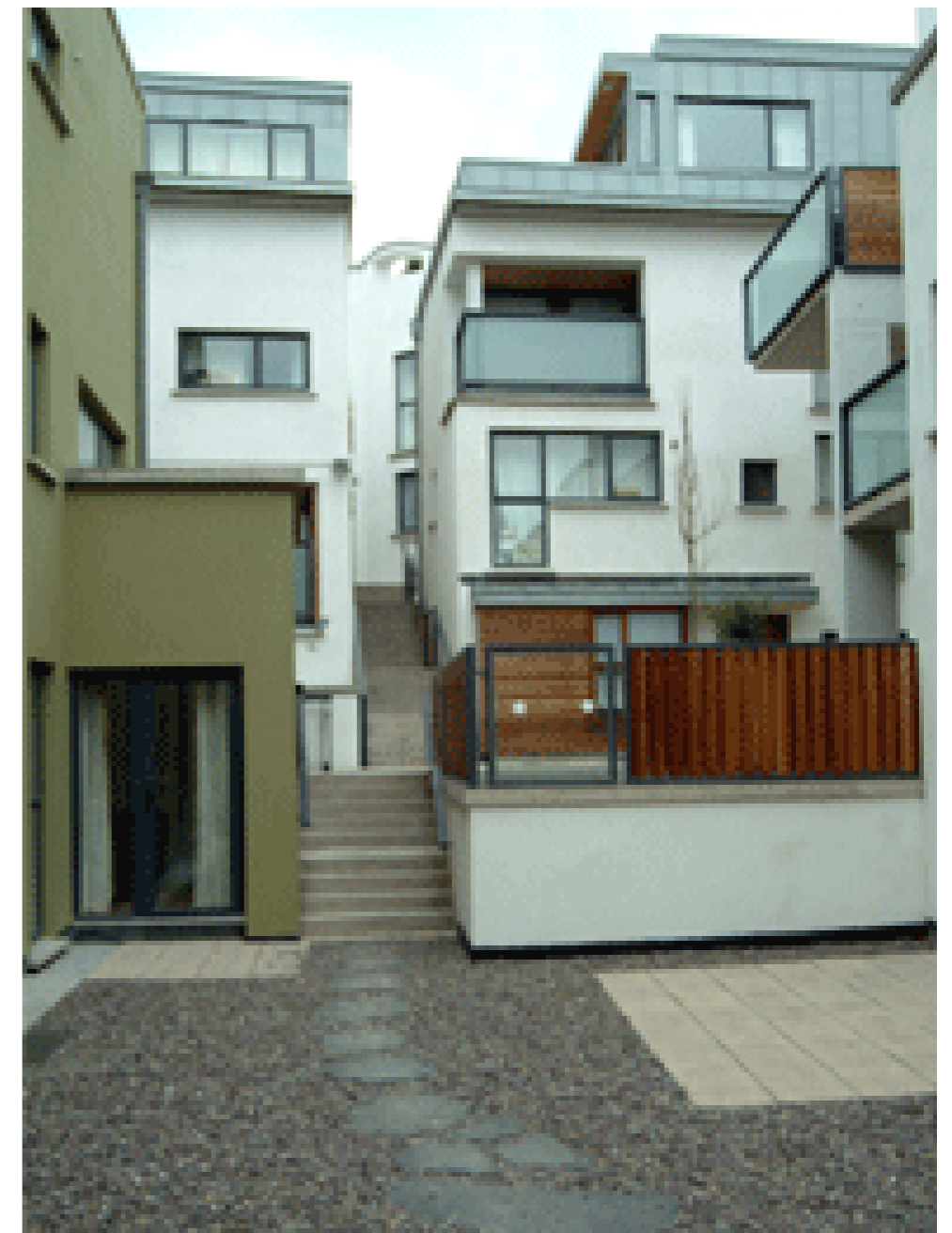
Fig 2.26 ACoppinger Court_Photo From DoEHLG Shaping The Future
