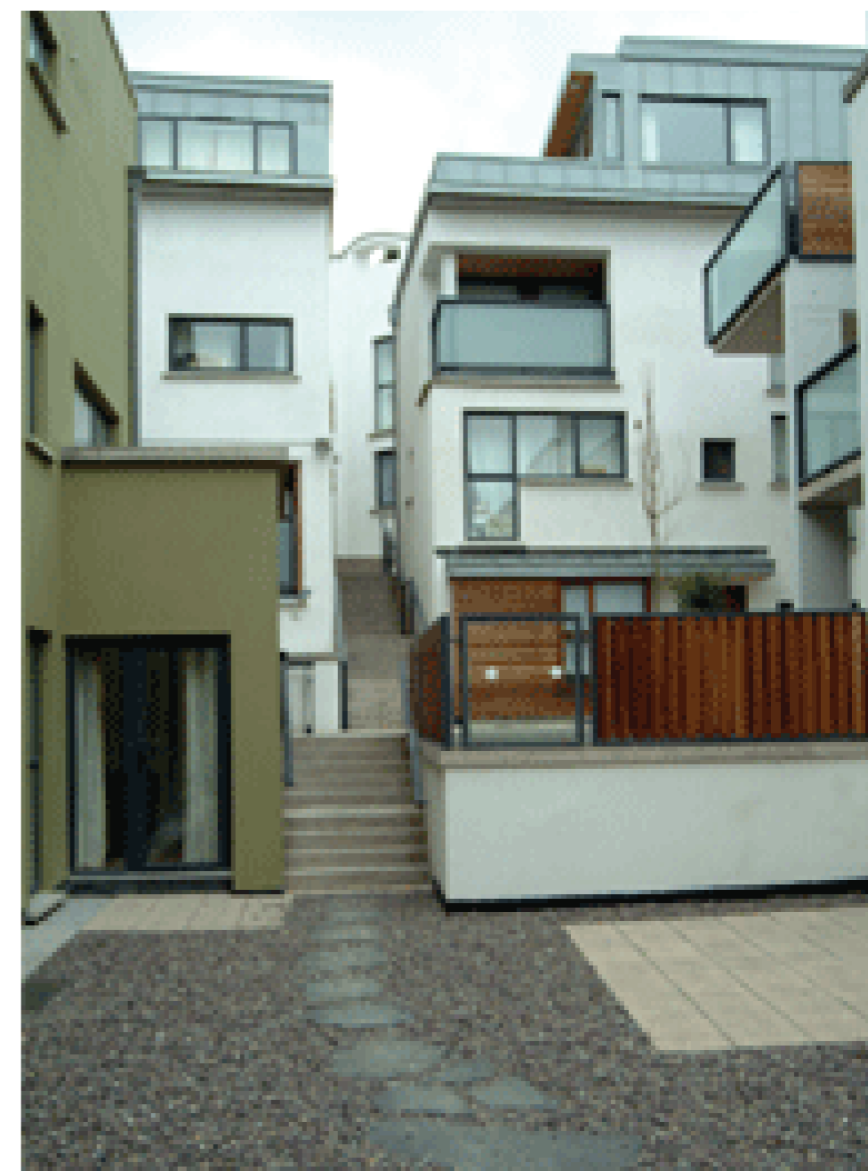
Fig 2.25 ACoppinger Court_Photo From DoEHLG Shaping The Future
