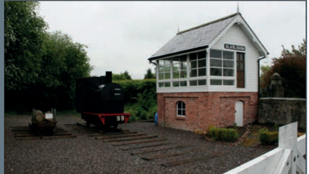
Glaslough Signal House renovation
