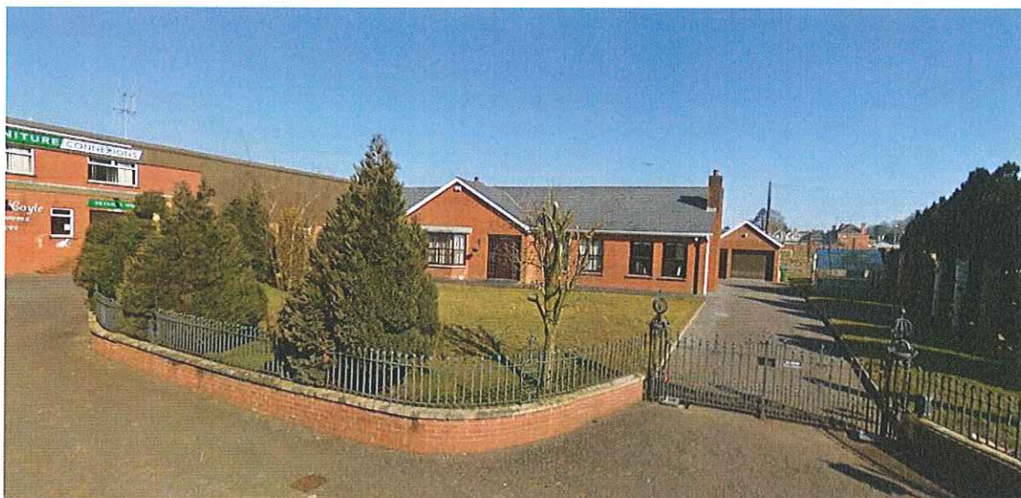
Figure 4.0 Street view of subject site, showing the interface with the adjacent office building
