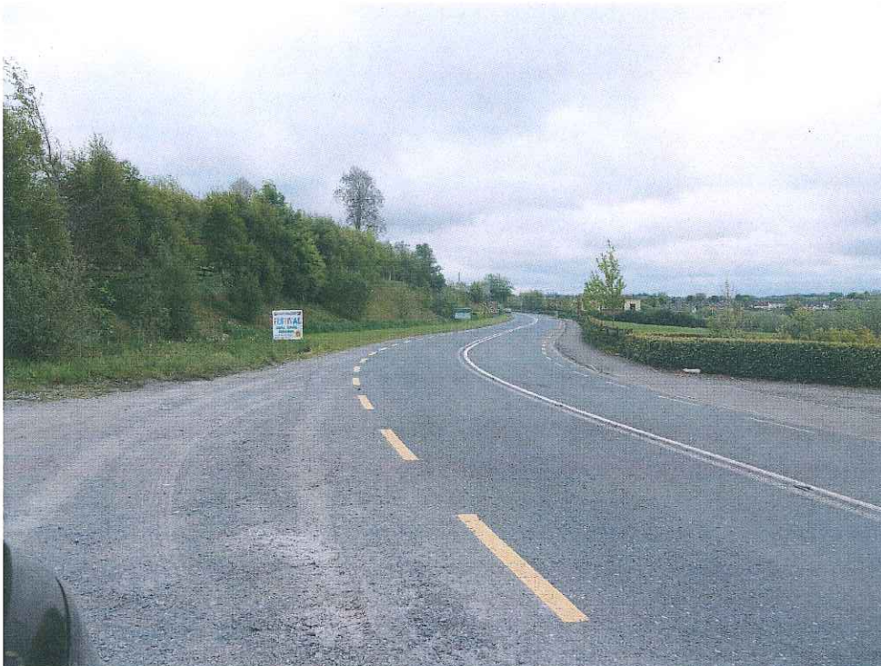
Suitable entrance onto public road in place.
