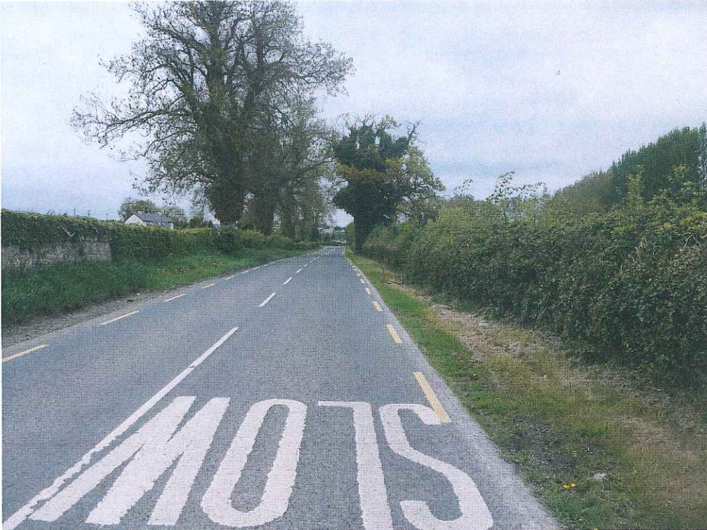
Suitable road margins can be maintained when providing sightline. View into Carrickmacross Public sewage mains on road.
