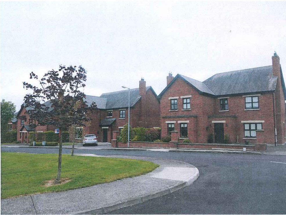
Standard of residence on this estate to match on new development
