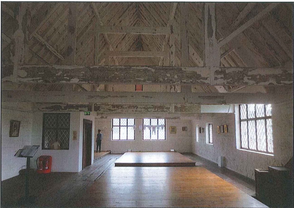
Plate 3 – The interior of one of the dormitories at Carrickmacross Workhouse located in the front western corner of the site, note the pine raised bedding area
