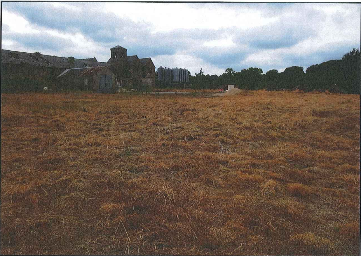
Plate 7 – The middle range of buildings on site at Carrickmacross Workhouse looking southwest, Carrickmacross, Co. Monaghan, note the precinct walls and rear range of buildings are now demolished
