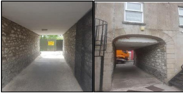
Figure 2: Images of subject building
