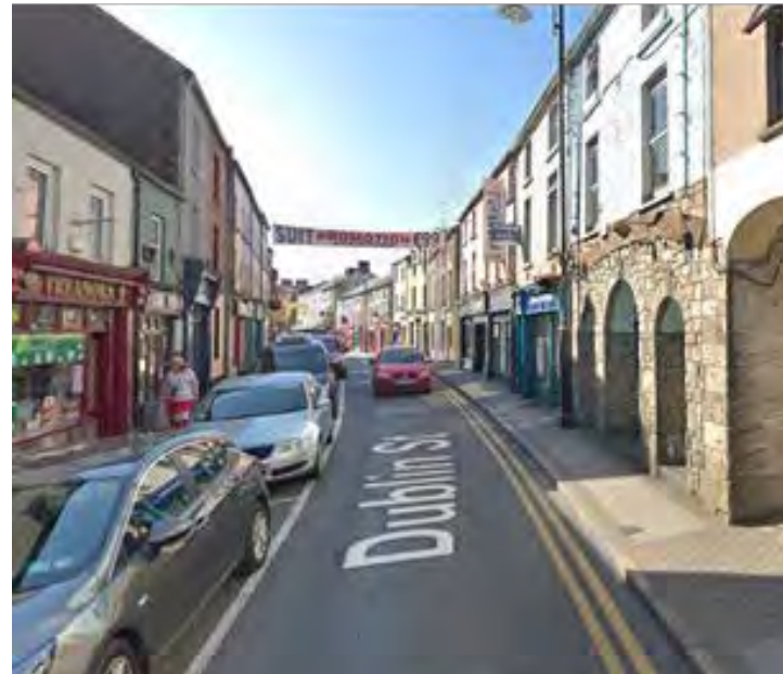
View of Dublin St From the East towards the West Google Street View
