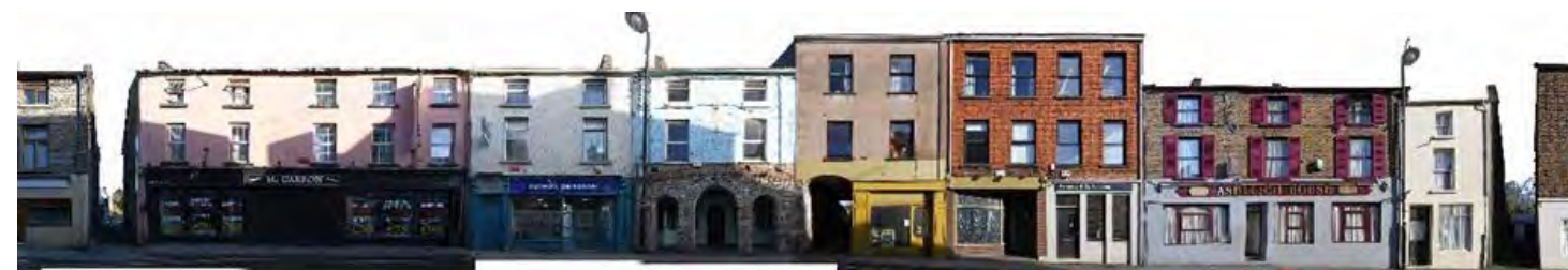
Elevation View of Existing Structures on Dublin Street—Dublin Street North
