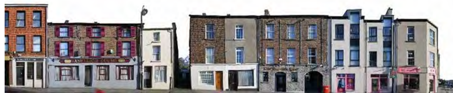
Elevation View of Existing Structures on Dublin Street—Dublin Street North
