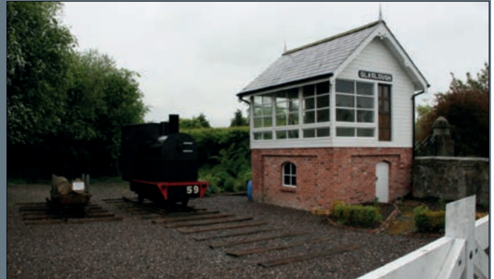
Glaslough Signal House renovation
