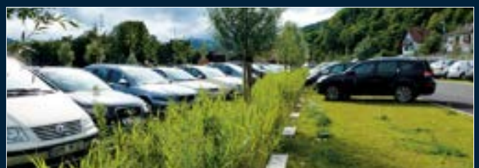
SUSTAINABLE URBAN DRAINAGE SYSTEM INCORPORATED INTO OVERSPILL CAR PARKING
