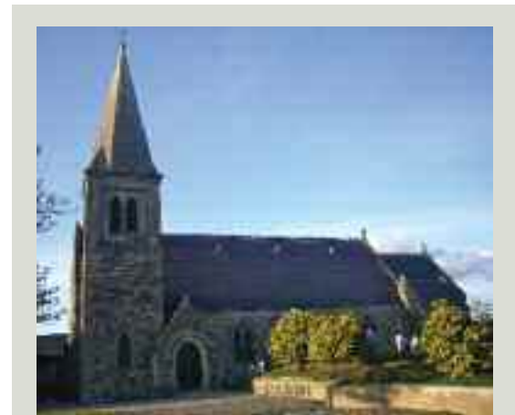
A nineteenth-century church with spire. The roof has been re-slatted and insulated and the walls re-pointed
