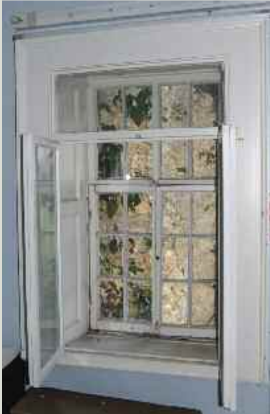
An Edwardian window with 1950s secondary glazing. The secondary glazing is chunky and does not match the original window profile and blocks light from the room. The position of the frame within the opening prevents the shutters from being used
