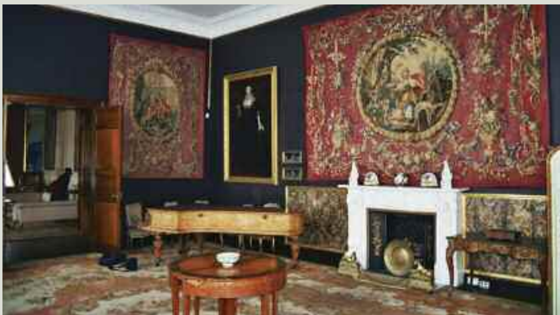
Leather linings and tapestries line the walls of this room and improve the thermal comfort of the occupants
