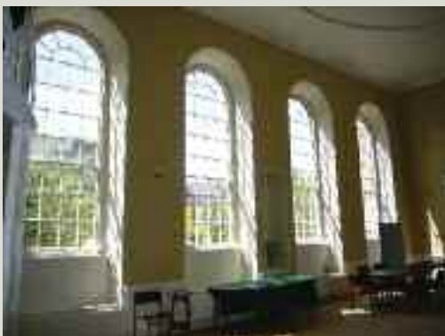
Tall, south-facing windows allow the main hall to be flooded with light and maximise solar gain
