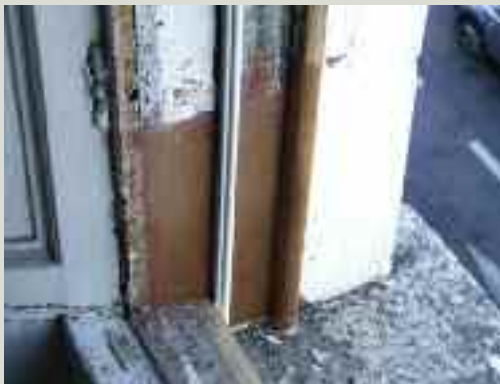
A repaired window frame with a replaced style and new parting bead. The timber sash frames have been temporarily removed
