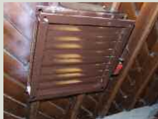
While re-slating, the opportunity was taken to put the original ceiling vents back into working order. The vents are mechanically controlled to allow the users to alter the amount of ventilation as required
