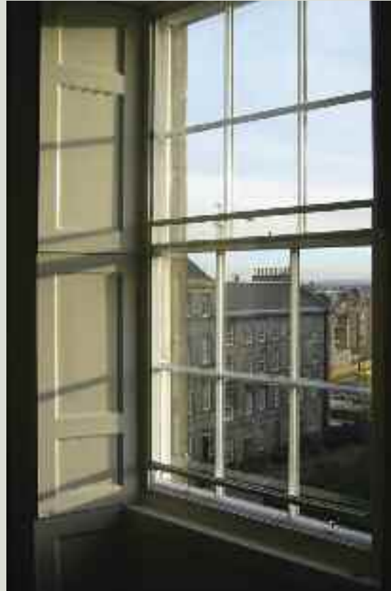
Carefully designed bespoke secondary glazing installed as part of Changeworks' Energy Heritage project (Image © Changeworks)
