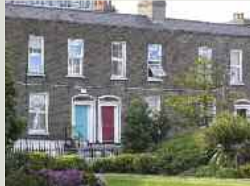
Terraced houses with replacement uPVC-framed windows. These windows are unsympathetic to the character of the houses; opening outward instead of sliding up and down, they disrupt the streetscape; the modern glass creates jarring reflections; while the thick frames contrast poorly with the elegant timber sections of the original sash windows
