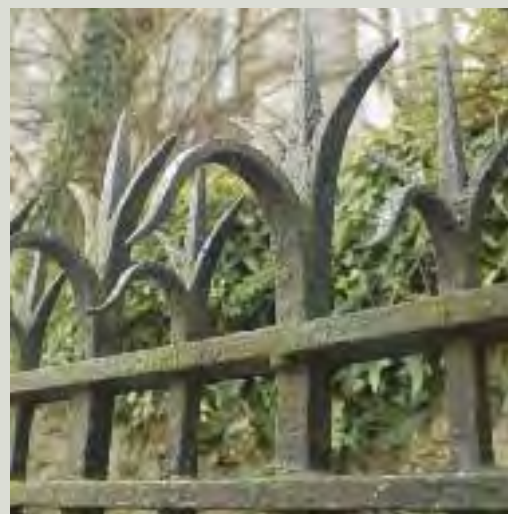
Note the pin just below the top rail of these wrought iron railings which would have been used to hold the rail in place during the assembly of the railings in situ
