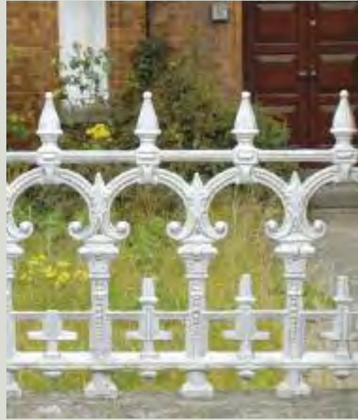
This design is typical of cast iron panels cast in repeating, identical sections. Patterns for railings such as these had to be designed so that there were no undercuts – it had to be possible to pull the pattern out of the sand mould without pulling away any of the sand (which would get trapped behind undercuts) in the process. Some panels have a taper from one side to the other which aided the removal of the pattern from the sand mould
