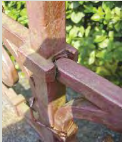
Cast iron railing panels were joined together by means of lugs and slotting systems such as the arrangement illustrated above
