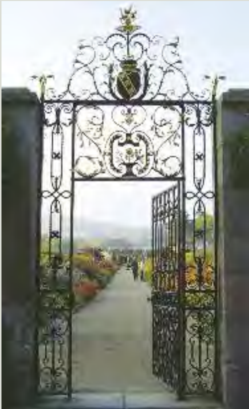
Delicate leaf-work is typical of wrought ironwork
