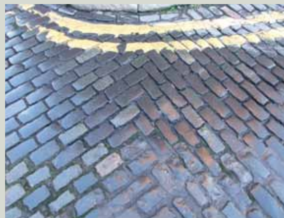
Examples of the skill and craftsmanship that is evident in traditional setted pavements
