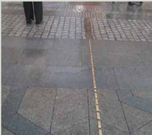
In some continental European cities, a system of guide strips is used to lead from crossing to crossing, which obviates the need for a tactile band across the footpath. In this example in Copenhagen, guide strips of elongated brass studs were retrofitted into modern paving
