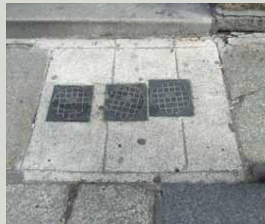
Access points set in concrete within a granite pavement in a manner not appropriate to the high-quality historic environment
