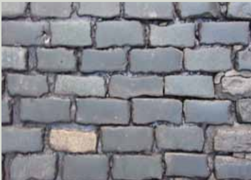
Setts poorly re-laid in sand-cement mortar with wide joints (above) giving the surface a very different appearance to an undisturbed historic surface (below) of tightly laid diorite setts
