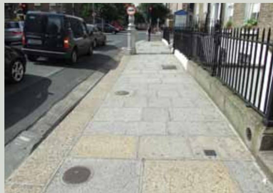
Replacement flags have been tooled to match the handmade texture of the historic ones
