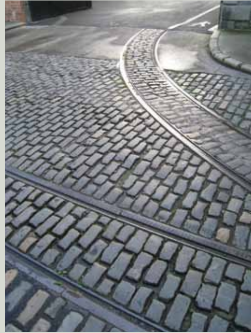
Redundant tram tracks at the Guinness Brewery
