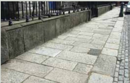
Granite flags at Mark Street, Dublin with wide kerbstones
