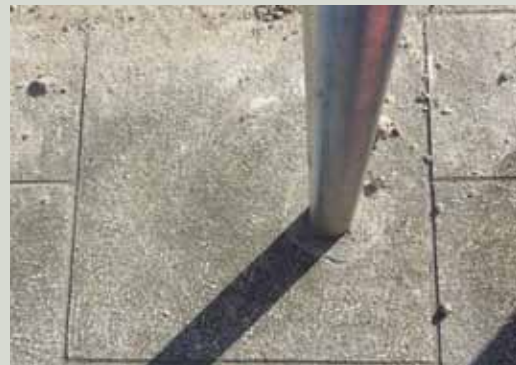
Good detail: a new flagstone is drilled to accommodate a signpost. Drilling a historic flagstone should be avoided in all but exceptional circumstances
