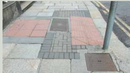
The unnecessary use of too many materials is unsightly, as is the ad-hoc placement of access covers
