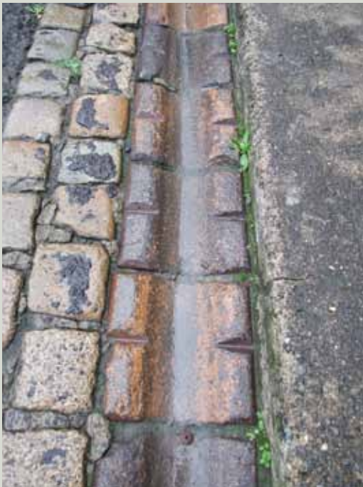
Formed fireclay gutter stones
