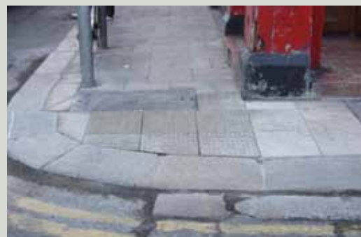
Tactile paving needs to provide a visual contrast but should follow the pattern and geometry of the existing paving
