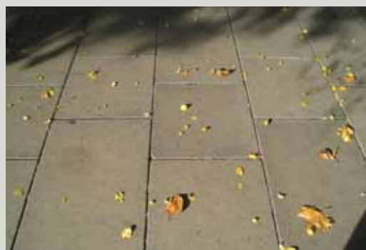
Concrete flags can be generous in size and laid in patterns similar to those used for granite or limestone flags. Good quality, smooth concrete flags wear well and can provide an appropriate setting to historic buildings
