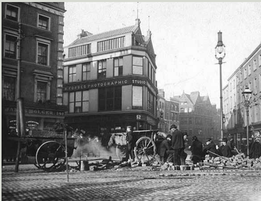
Road repair works underway on Saint Stephen's Green at the top of Grafton Street, Dublin c.1900 (Lawrence Collection, image courtesy of the National Library of Ireland)
