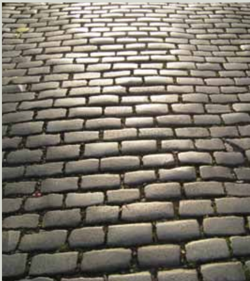
Evenly worn diorite setts at John's Lane West, a rare finish, full of character, which is impossible to recreate with new materials
