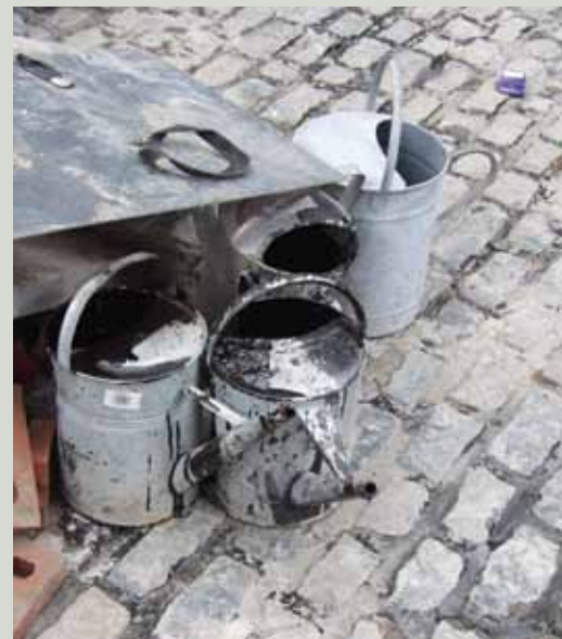
Cans for tar grouting
