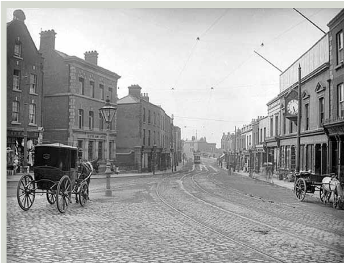
Main Street, Blackrock, County Dublin with a setted street incorporating tram tracks (Lawrence Collection, image courtesy of the National Library of Ireland)
