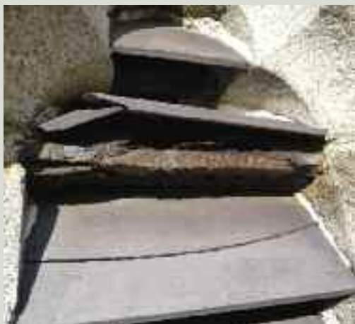
Embedded metal tie bars in this bell tower corroded and expanded, causing fractures in adjacent granite and slate louvres. Part of the repair solution involved installing a cathodic protection system to reduce the corrosion rate of the embedded ironwork
