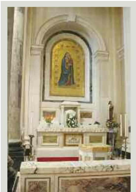
This richly decorated Neoclassical baptistry is separated from the body of the church by Connemara marble columns, which have polished black limestone plinths. The Carrara marble-clad niche houses an Italian gold-leaf mosaic panel
