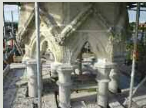
This Bath stone turret, which is also a bell-tower, is in a highly exposed location. Several stones cracked due to rusted cramps and the poor condition was exacerbated by previous misguided cementitious repair. New stainless steel collars and ties were fitted and the turret was repointed
