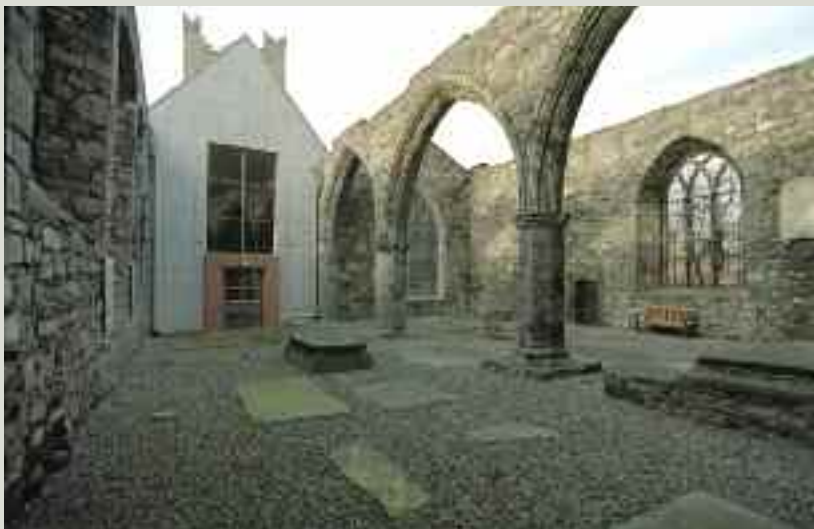
The medieval chapel of Saint Anne at Saint Audoen's Church of Ireland, Dublin was converted to a visitor centre in 2000. The work included re-roofing the chapel and the construction of a new east gable wall. The wall is a spare, modern intervention in a highly sensitive location facing onto the former Portlester Chapel and chancel of the medieval church
