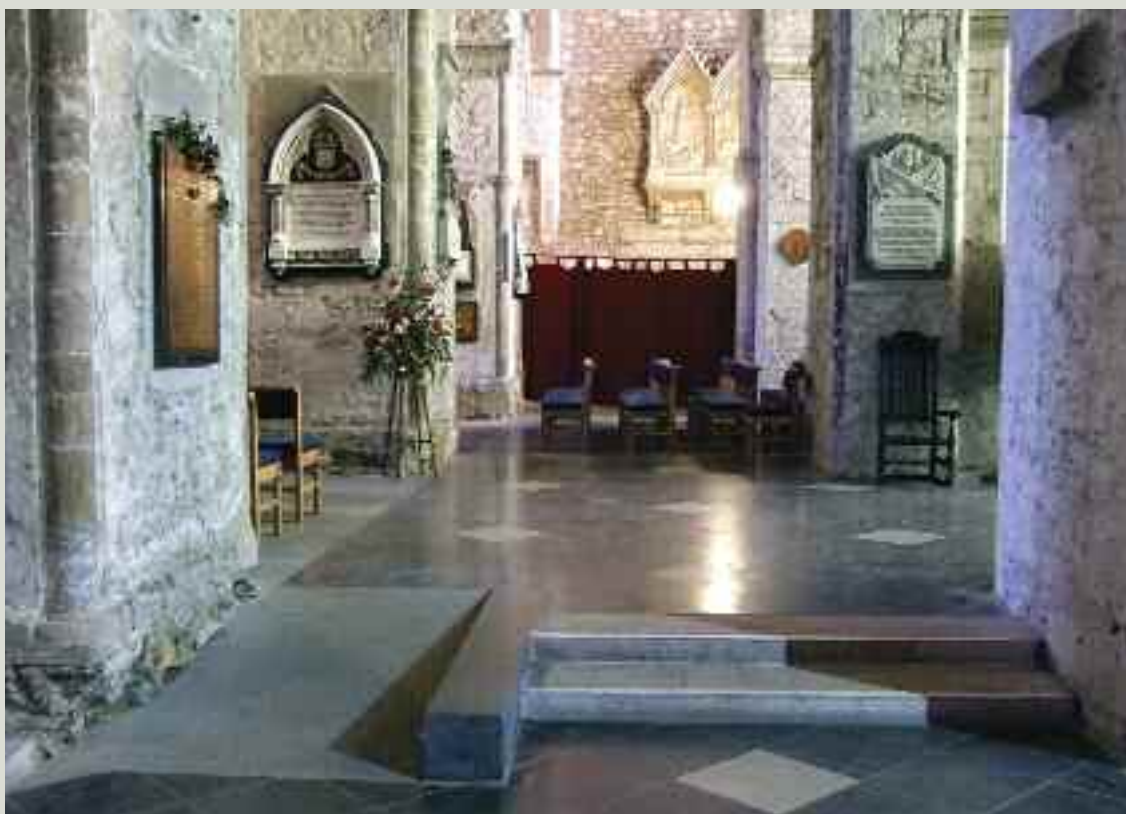
Improving access where there are several changes of floor level within a church requires careful consideration. Where the church is a medieval structure, there is the possibility of burials beneath the nave which preclude lowering of the floor level. Ideally, the improvement of access should be an integrated part of an overall conservation strategy
