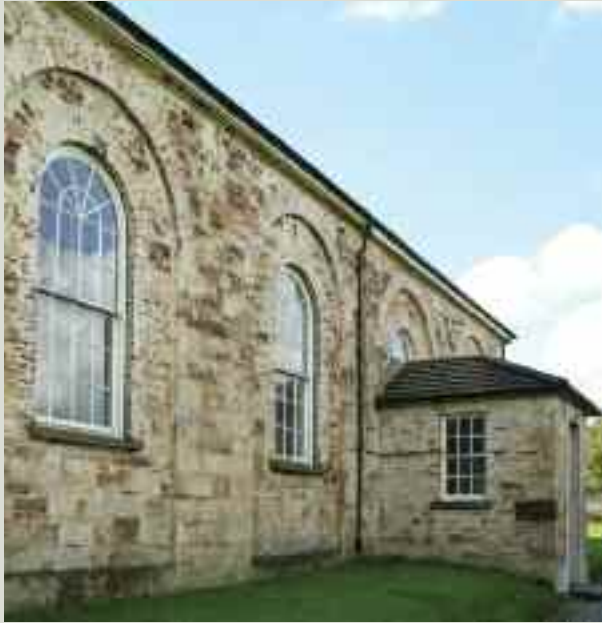
The Society of Friends built this elegant Neoclassical meeting house in Cahir, County Tipperary in 1833. In 1881, it became a Presbyterian church and remains so today
