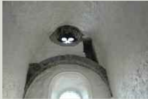
The cement plaster on this Romanesque church, which was damaging the stonework and associated timbers, was carefully removed and replaced with a soft lime plaster
