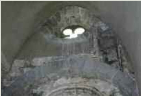
The cement plaster on this Romanesque church, which was damaging the stonework and associated timbers, was carefully removed and replaced with a soft lime plaster
