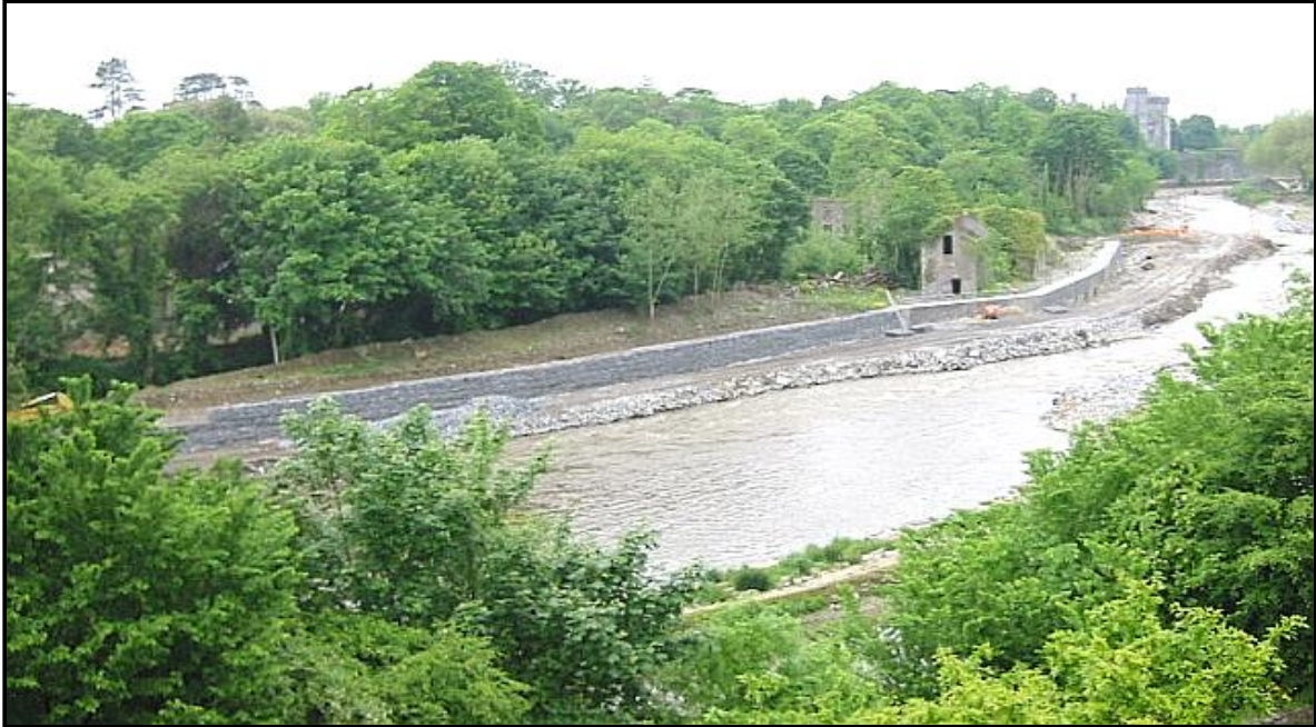
Figure F.3: River Widening (During Construction)
