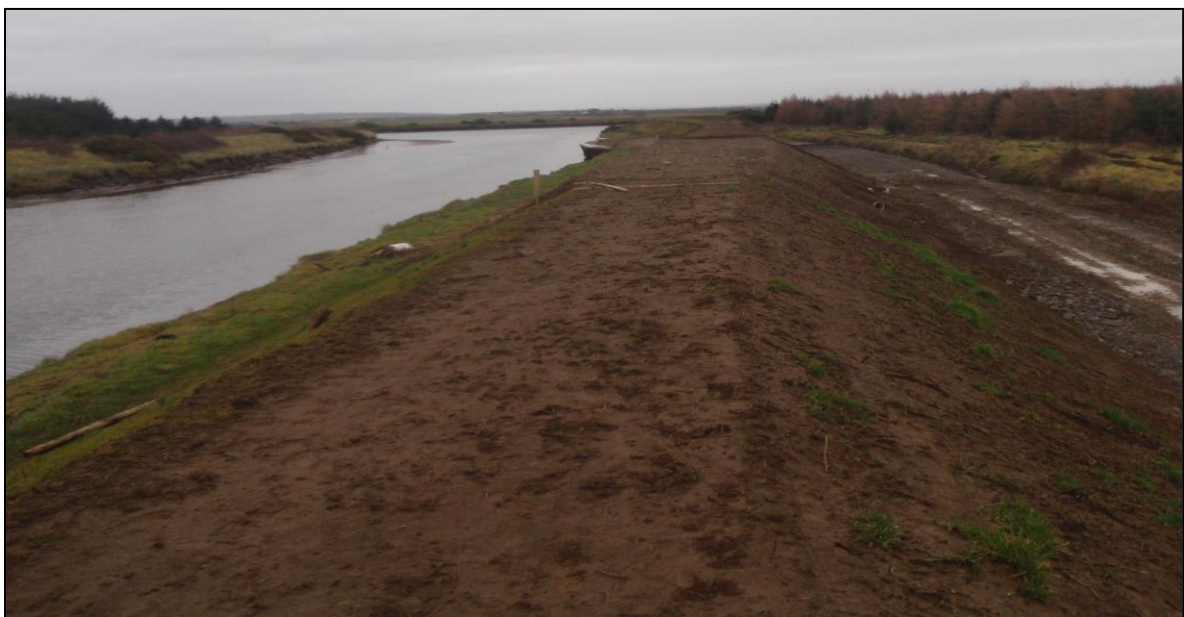
Figure F.2: Flood Defence Embankment (During Construction / Maintenance)
