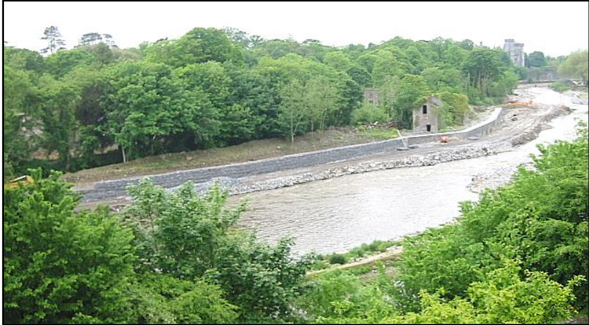
Figure F.3: River Widening (During Construction)
