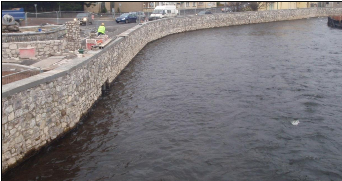
Figure F.1: Flood Defence Wall
