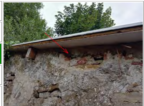
Photo No. 3 - Roof tile packer below modern corrugated metal roof - north side high elevation
