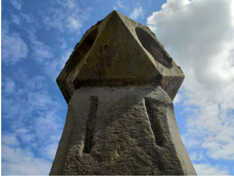
Detail of later augmentation for gas lantern and/or public notice mount (left) and chasing for gas pipework (right)
