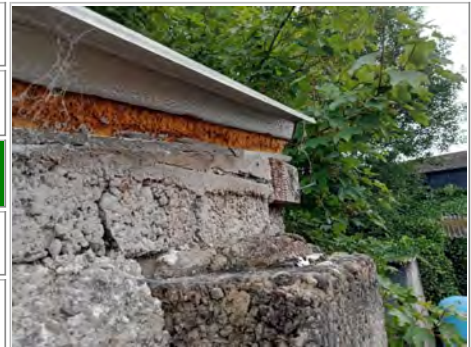
Photo No. 2 - Roof tile packers below modern corrugated metal roof - high level east elevation
