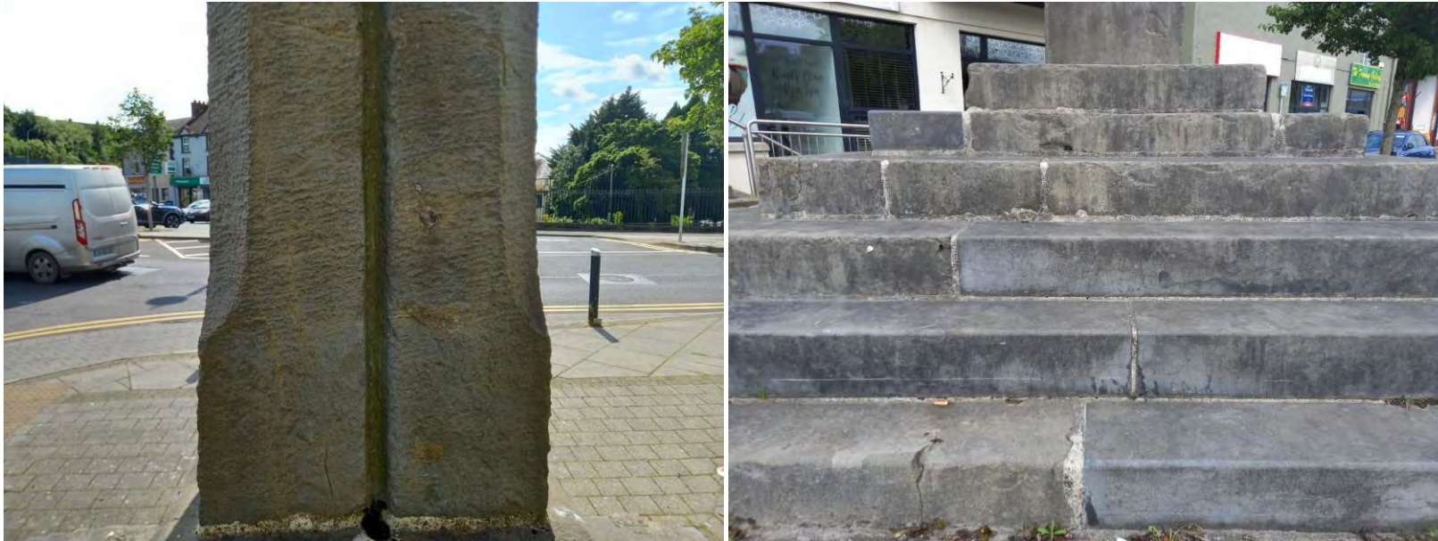
Detail of cut chasing for gas pipework (left) and limestone step conservation and replacement works undertaken in 2011 (right)
