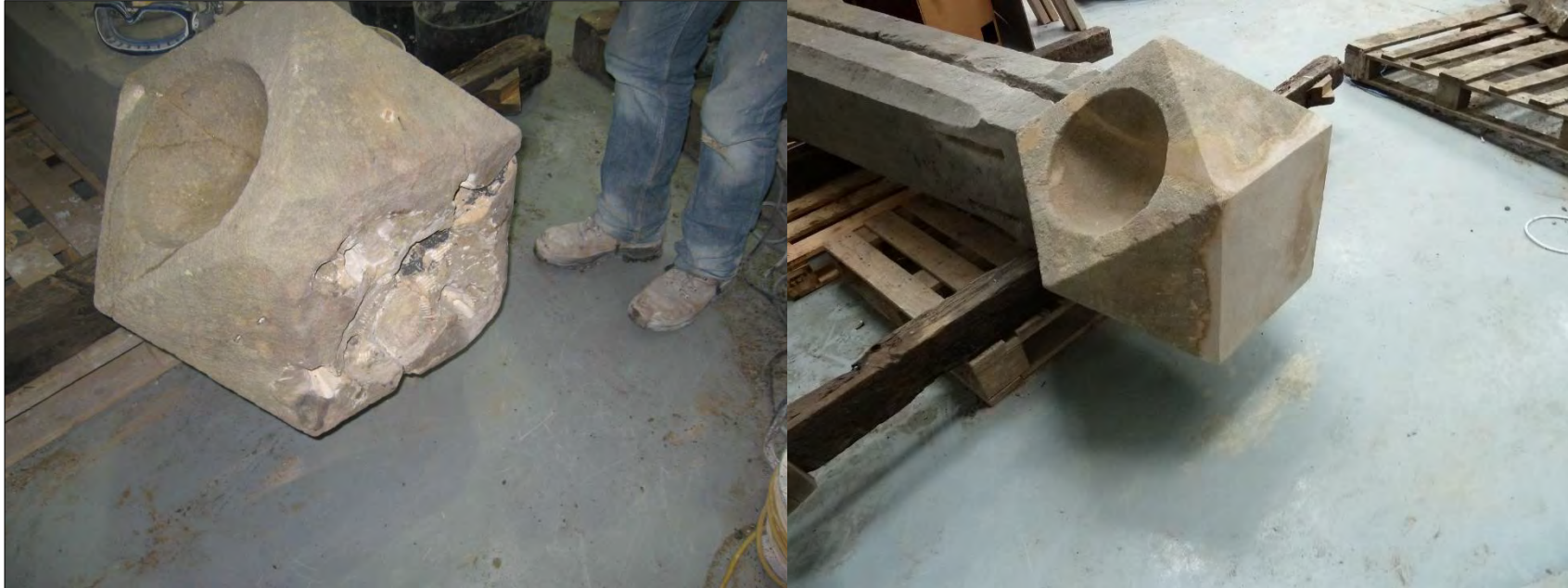
Figure 6 Evidence of gauging out of the sandstone sundial (left) to accommodate a gas lantern in the later nineteenth century. This was repaired (infilled) (right) and the sundial corrected to its original upright functional position atop the shaft, as part of 2011 conservation works. (Image source: D. Nolan, 2011) 6
