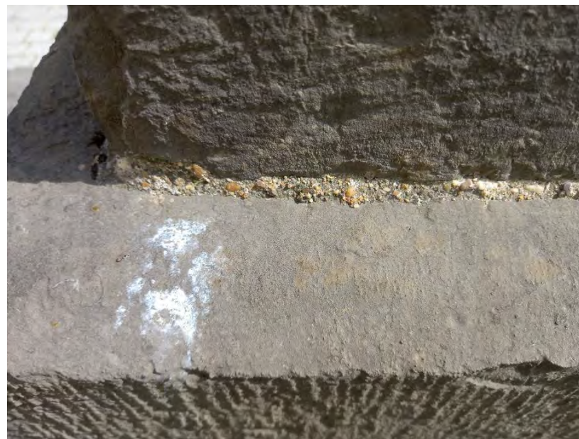
Detail of plinth repair works (left) and mortar detail (right) undertaken 2011
