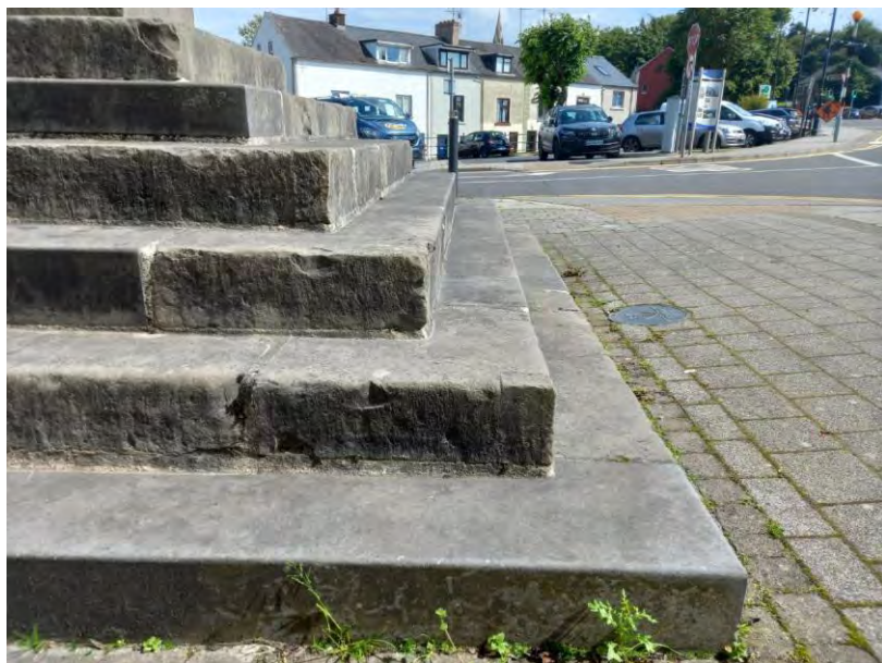
Detail of limestone step repairs and replacement conservation works (undertaken 2011)
