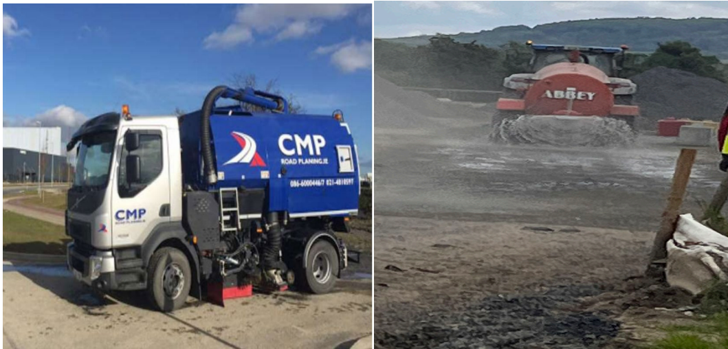
Figure 4.3: Dust suppression methods using road sweeper and water bowser
