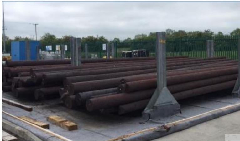
Figure 2-4: Placement of poles over absorbent matting contained within stanchions
