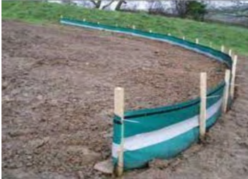
Figure 3-2 Example of silt fence
