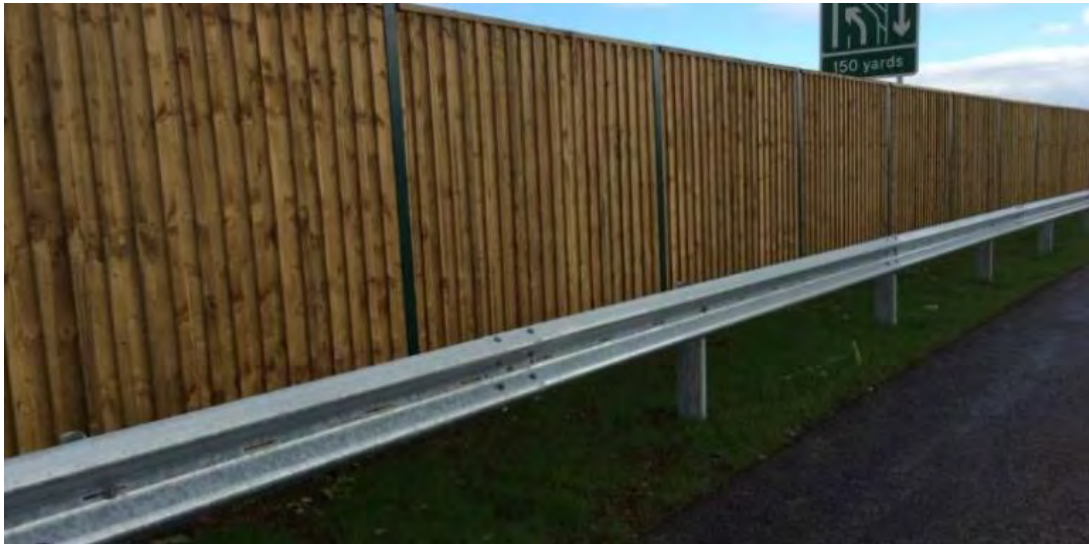
Figure 3-1 Example of noise barrier fence
