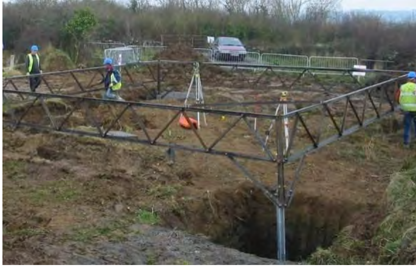
Figure 4-2 – Traditional ESB stub setting template
