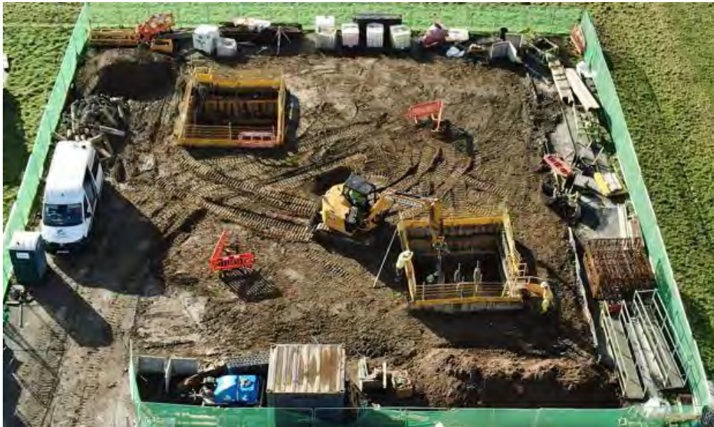
Figure 6-8 – Mini pile foundation stage: Works at legs 2 and 4
