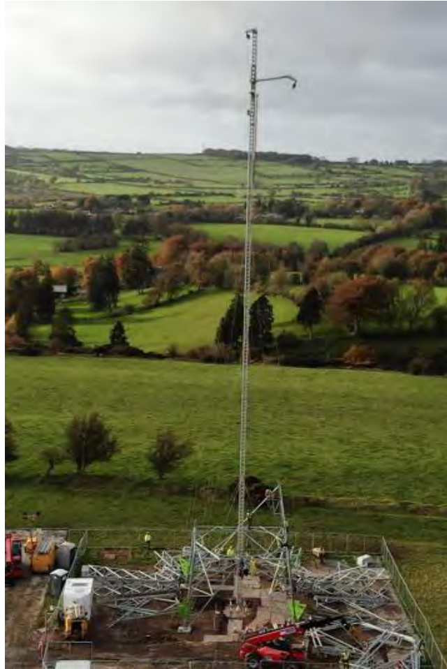
Figure 6-4 – Gin pole erected
