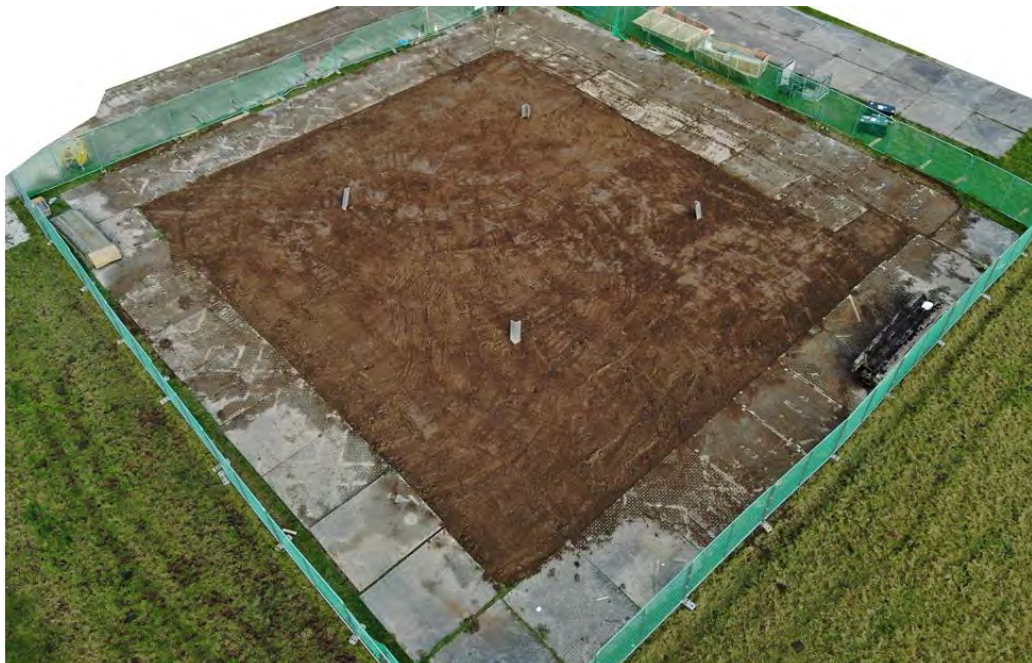
Figure 6-2 – Tower stubbed and surplus spoil graded within the works area
