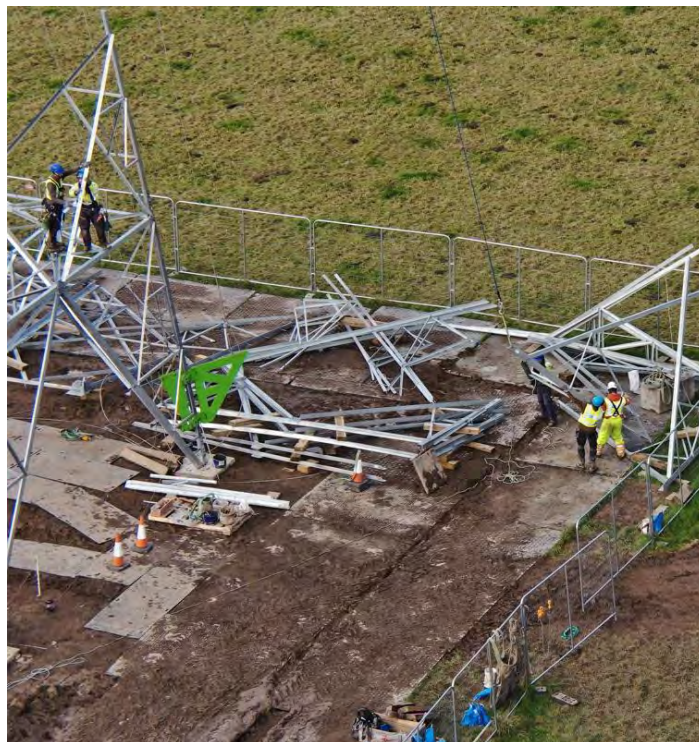
Figure 6-5 – Preparation of tower section for lifting
